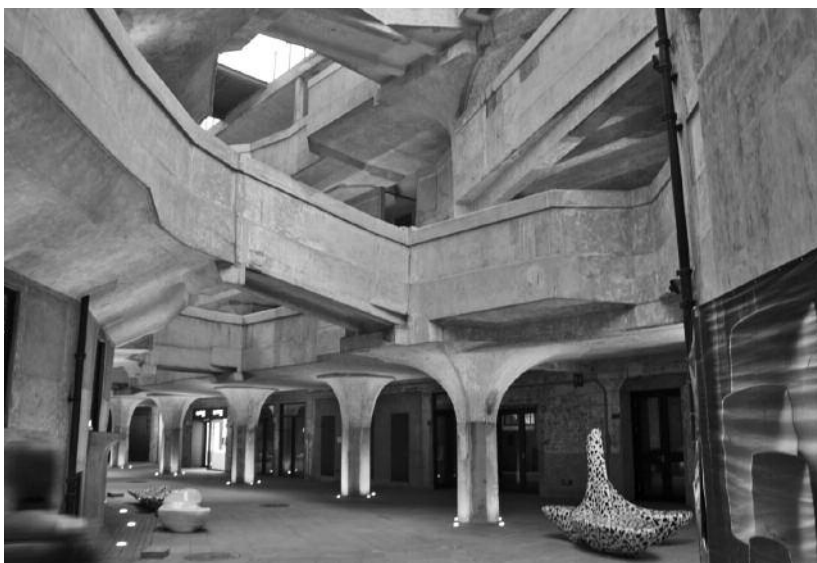
1933 Old Millfun – the former slaughter house after restoration.
