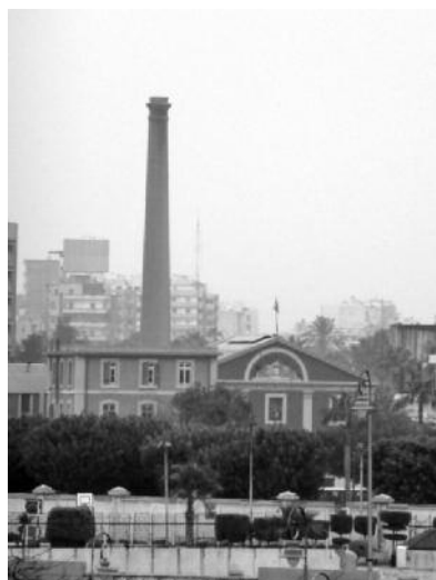
Chimney and building of Alexandria Water Company, built around 1886, standing gracefully in the urban landscape of Alexandria.
