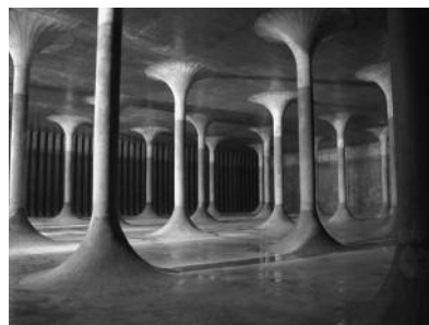
Reinforced concrete pillars in the underground cistern of the Budapest Waterworks on the Gellért Hill from 1980.
