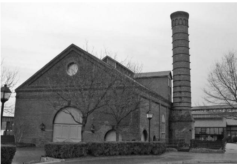
Figure 1: The 1861 Tredegar's gun foundry building that has been restored and now is home to the American Civil War Center
