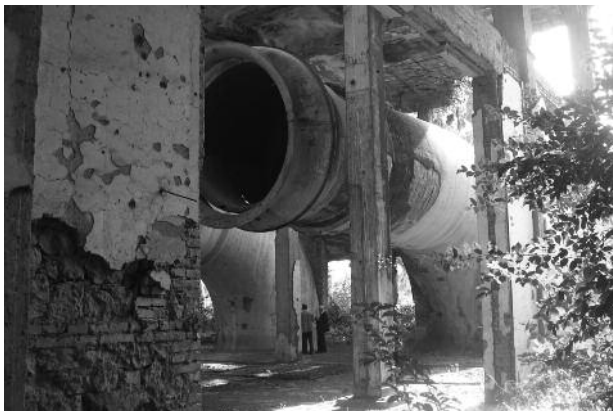
Actual view of the horizontal wind galleries.
