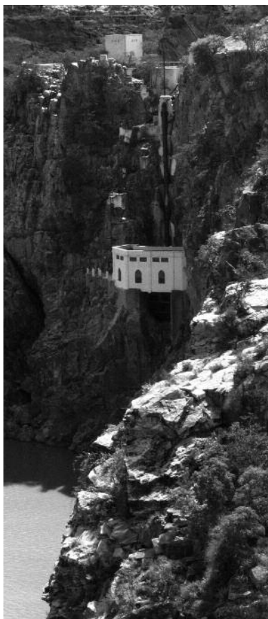
The impressive Angiquinho hydroelectric power plant in Pedra.
