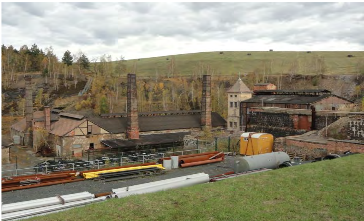
Muldenhütte Smelting Works near Freiberg, Germany
