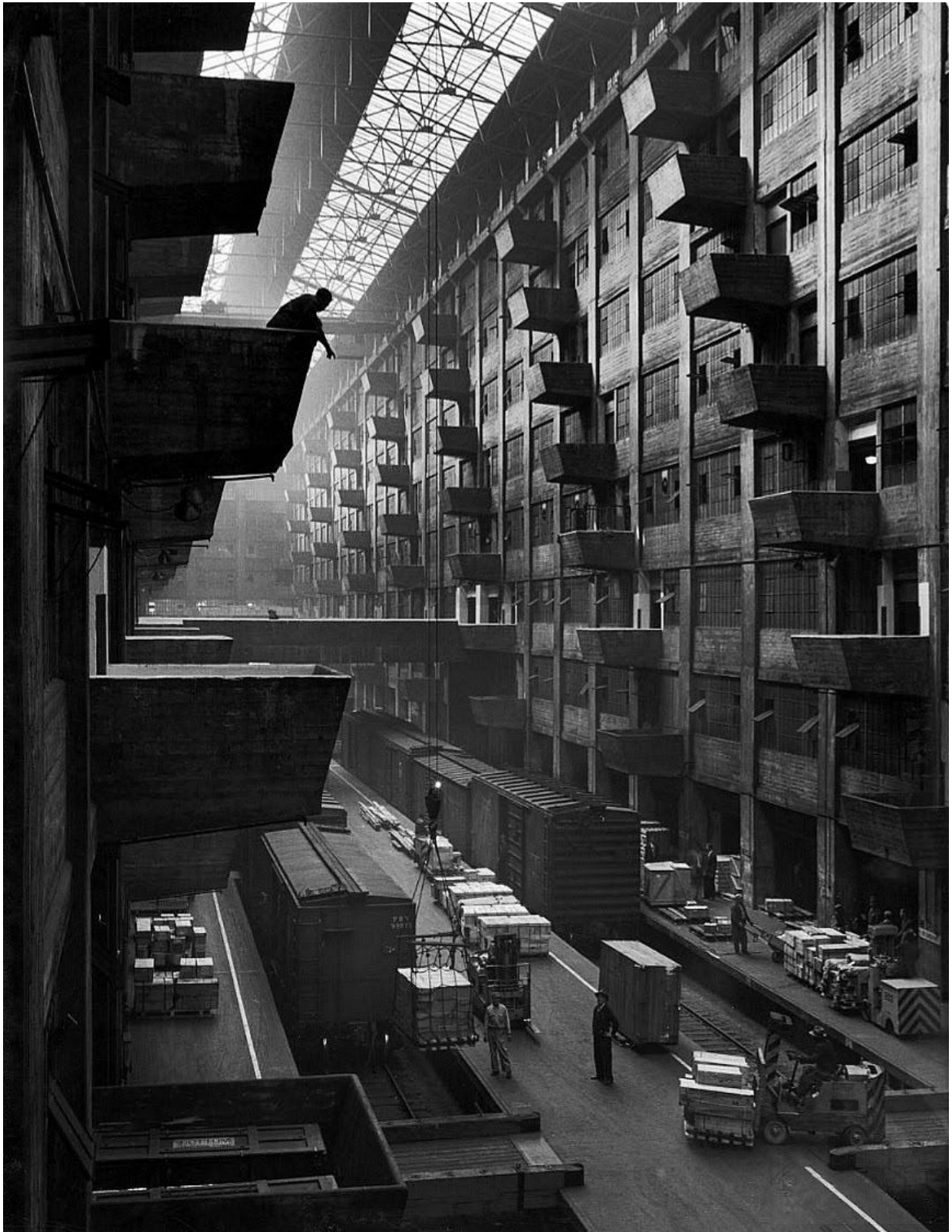
1948 photograph for Life Magazine inside the Brooklyn Army Terminal Building B. The suspended ceiling crane travelled the length of the building beneath the glazed atrium roof, raising and lowering freight between the projecting, staggered balcony loading docks and the railway cars which were driven directly inside the building.
