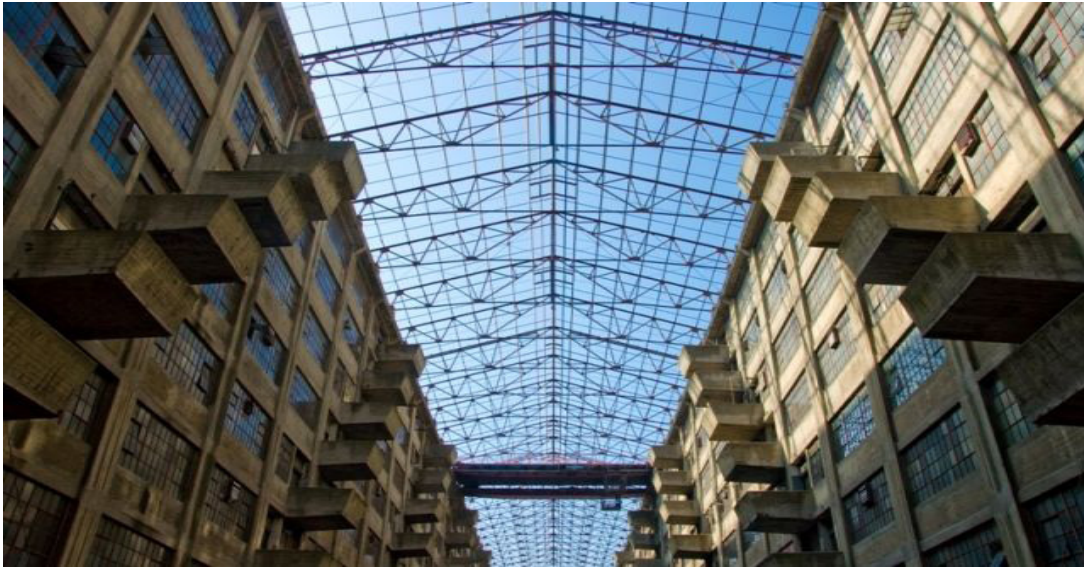
The magnificent sky-lit atrium in Building B; one of the most dramatic early twentieth century interiors in the US.
