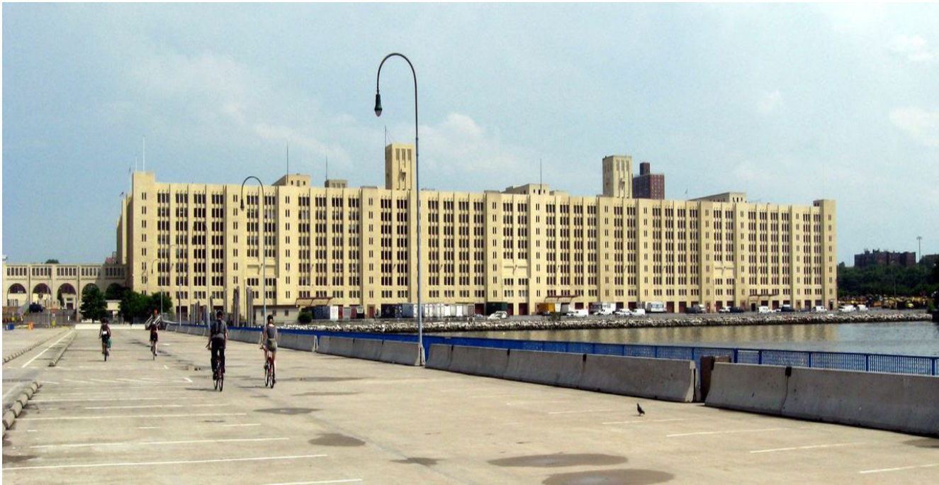
The phased refurbishment over twenty years of the two enormous warehouse buildings by the New York City Economic Development Corporation has attracted business and light manufacturing and kick-started economic regeneration along the waterfront.
