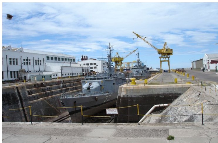
Dry dock in use during 2006. At present time, Argentinian Navy ships and foreign merchant vessels are repaired here.
