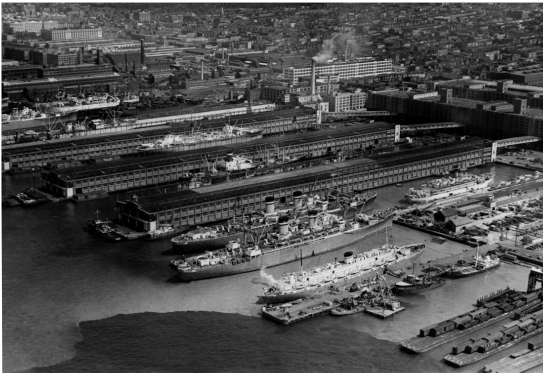
Aerial view of the Brooklyn Army Terminal during World War II - its busiest period of operation. Sky bridges and rail lines connected the two 980ft long terminal buildings to enormous sheds straddling each of the four piers, enabling the rapid transfer of goods, equipment and troops between land and sea.
