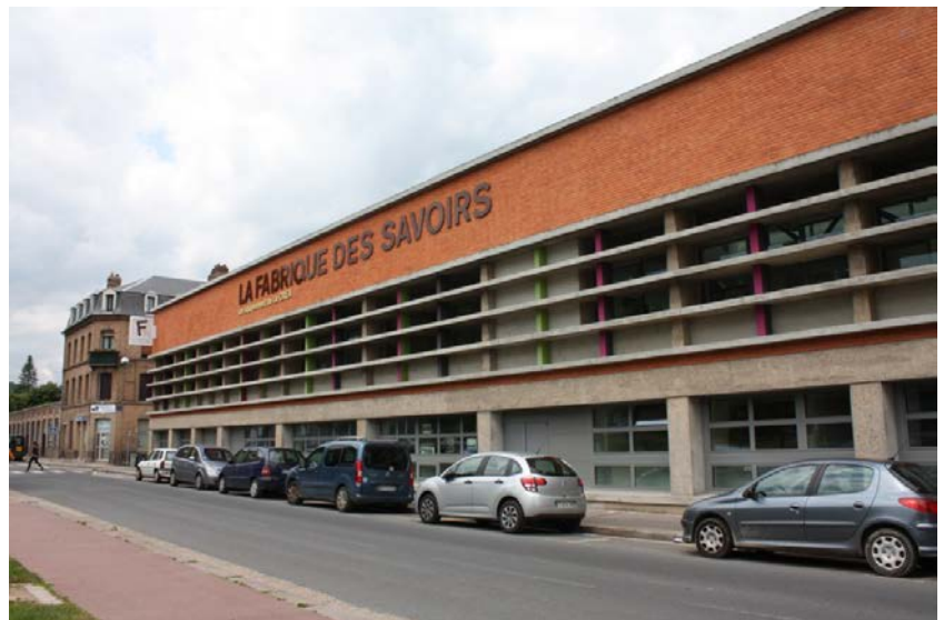
La Fabrique des Savoirs. The museum opened in a part of the former Blin & Blin manufactory.
