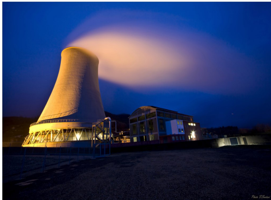
Geothermal power plant Sasso 2
