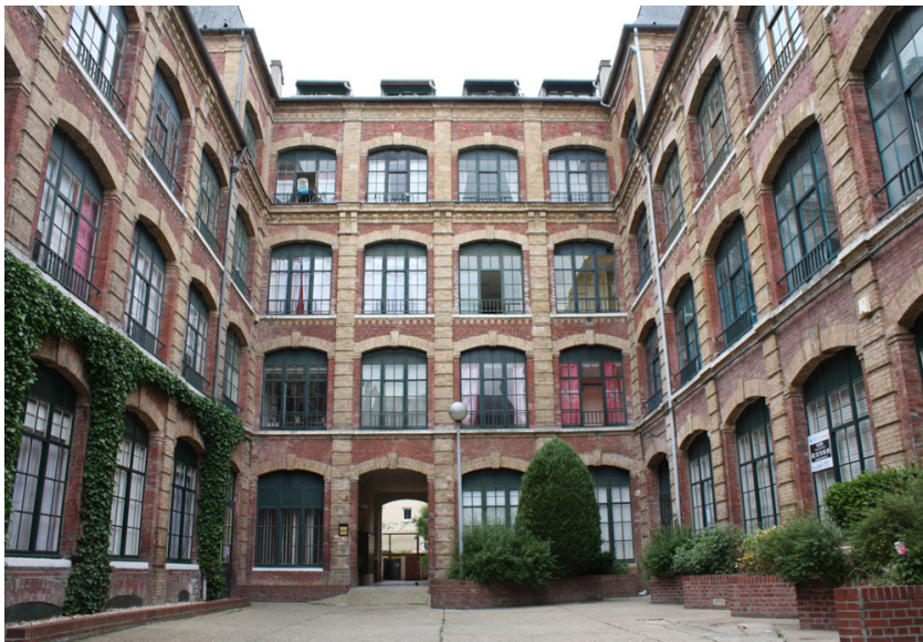
Nivert & Bourgeois factory. Factory built in the 1860s for finishing processes, acquired after the First World War by the Nivert & Bourgeois firm. The surviving buildings are arranged in a U-shape around a courtyard are only a third of the original ones. They offer office space today for some of the city's medical cabinets and law firms.
