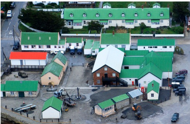
The group of historic dockyard buildings in Stanley that form the new museum.
