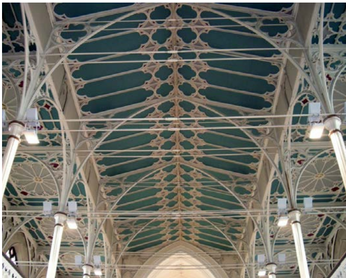
The cast-iron interior of St George's Church, Everton, 1813-14, designed by J M Gandy, John Cragg and - possibly - Thomas Rickman with castings manufactured by the Mersey Iron Foundry.
