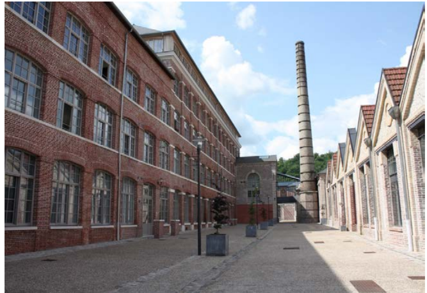
Gasse & Canthelou factory. Situated in the centre of the city, this factory specialized in weaving and finishing of woollen cloth. A 1842 timber-framed building with an 1882 metal framed addition and a new north-lit weaving shed added in 1918. The factory has been converted into housing and was awarded the Auguste Perret Prize in 2010.
