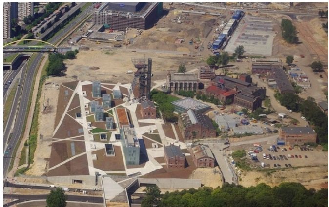
Aerial view of the Area of Culture with the surface building of the former mine.
