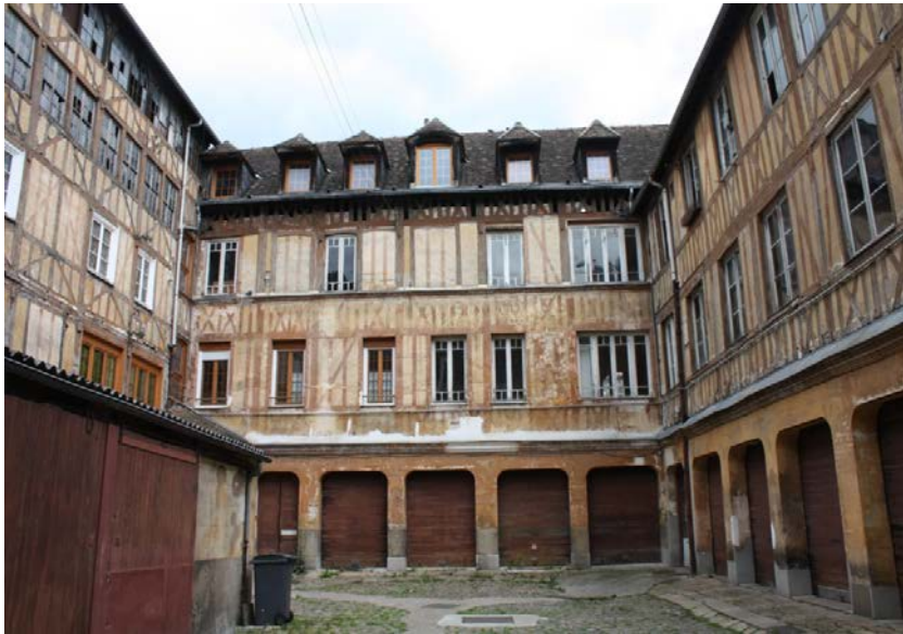
Charles Houillier Manufactory. A courtyard of three timber-framed workshops from the second half of the 17th century, rebuilt and raised a floor during the 19th century, and transformed some time ago into housing.
