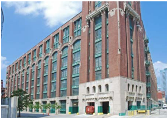
Chicago's Lakeside Press Building was built between 1912 and 1929 and is now known as the Lakeside Technology Center. This handsome daylight factory with Art Deco decoration was designed by Howard Van Doren Shaw.
