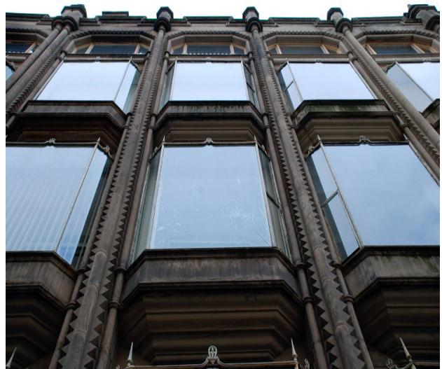
Oriol Chambers, 1864, by Liverpool architect Peter Ellis, an iron-framed office building, described by Nikolaus Pevsner in 1969 as 'one of the most remarkable buildings of its date in Europe' and by Charles Reilly as a 'cellular habitation for the human insect'. The facades are almost wholly of glass, the cantilevered oriels designed to capture light in the narrow confines of the city
