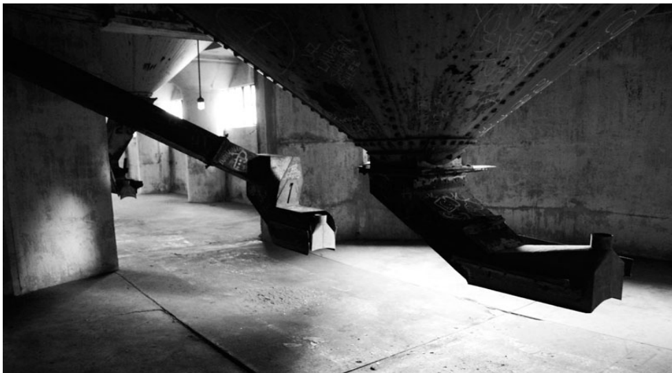
Grain hoppers inside Marine 'A' Elevator (1925)
