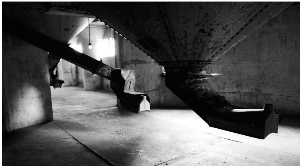
Grain hoppers inside Marine 'A' Elevator (1925)
