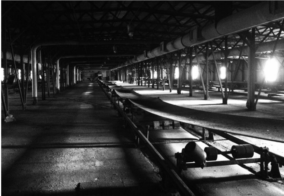
Horizontal conveyor on the bin deck inside the Perot Malting Elevator (1907)
