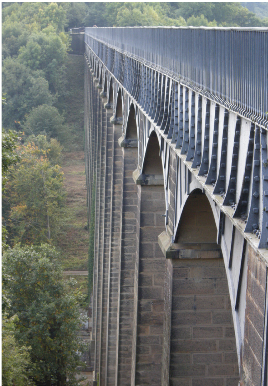
The greatest heritage asset of the CRT is Pontcysyllte Aqueduct; restored by BWB for the bicentenary of its completion in 1805. It was designed by Thomas Telford and William Jessop and consists of a cast-iron trough 307m long carrying the Llangollen Canal 38m above the River Dee. Inscribed on the World Heritage List in 2009.
