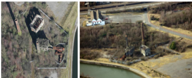
The two surviving engine sheds and rolling machinery at the Hafod Copper Works site.
