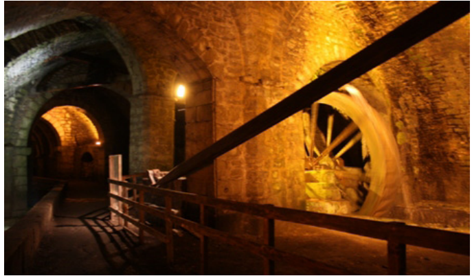
Salins-les-Bains. The restored underground galleries and pumping mechanism.
