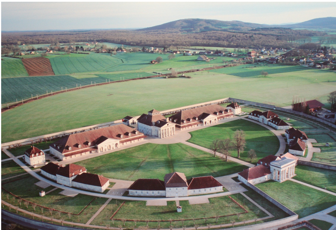
Nine radiating paths divide the works and converge on the central director's house, the 'temple of surveillance'. On either side are the two main industrial buildings or 'bernes', housing the pans. Around the circumference are various ancillary buildings, a forge, cooperage and workers' dwellings.
