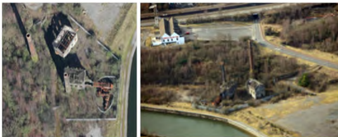
The two surviving engine sheds and rolling machinery at the Hafod Copper Works site.
