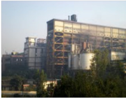
The Rajghat Thermal Power Plant in Delhi, India.
