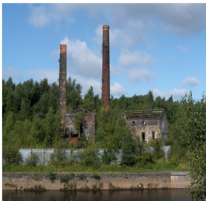
Last vestiges of the historic Hafod copperworks, Lower Swansea Valley, Wales.
