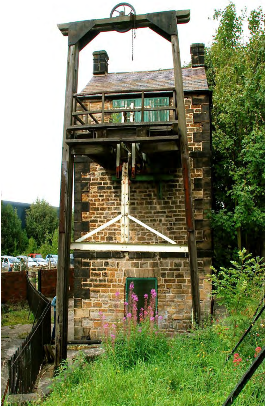
The Elsecar engine was built in 1795, draining water from Elsecar New Colliery until 1923 and remained in working order until the 1950s
