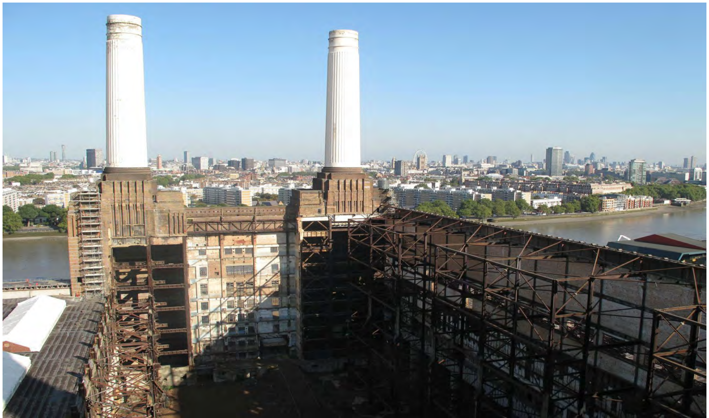
The view into the gutted interior of the former generating hall and two of the four chimneys, in 2009.
