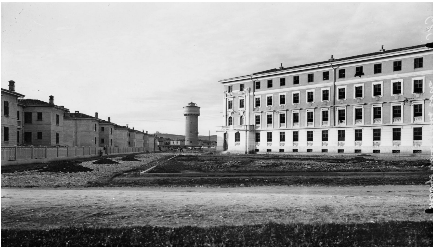
The new museum occupies the Albergo Operai, the Workers' Hostel.
