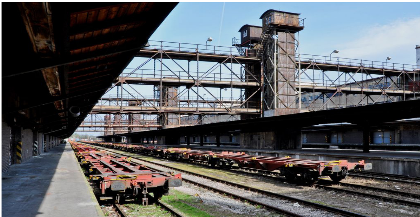
Between the two wings of the Žižkov Freight Station (1931-1936), Prague. Road access was from the outside of both warehouse ranges.
