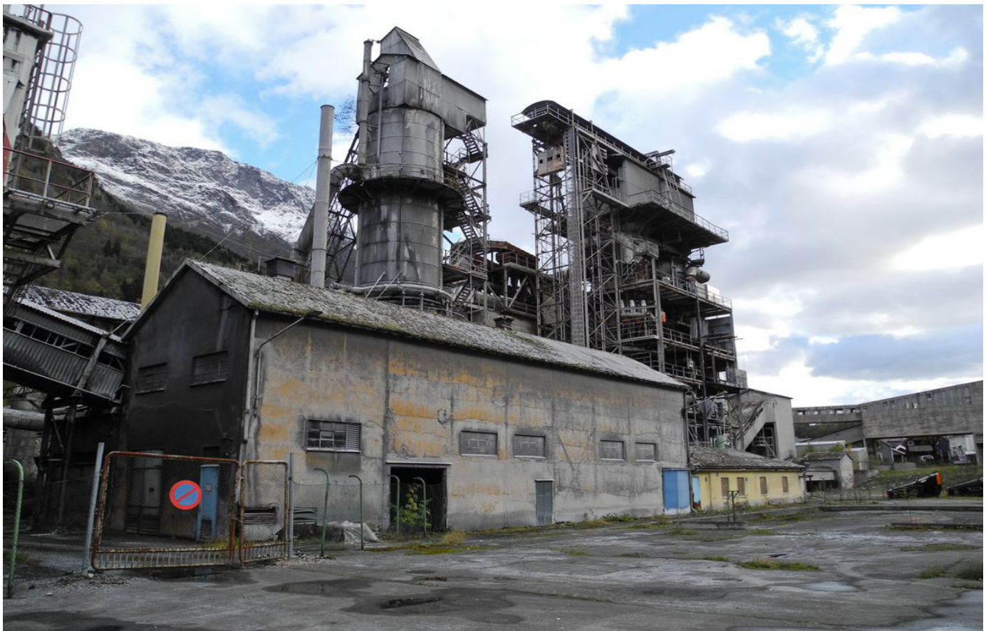
The lime kilns and coke driers at Odda smelteverk in October 2011.
