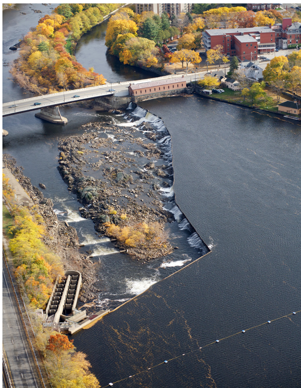
The Pawtucket Dam dam is in many ways the centerpiece of the historic industrial complex at Lowell as well as a key to the interpretive scheme in the National Park. Photo © James Higgins.
