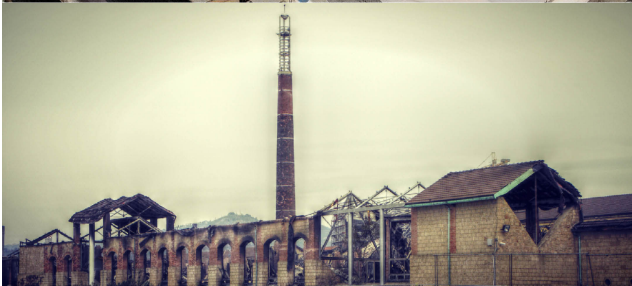
The Naples Science City before and after the arson attack.
