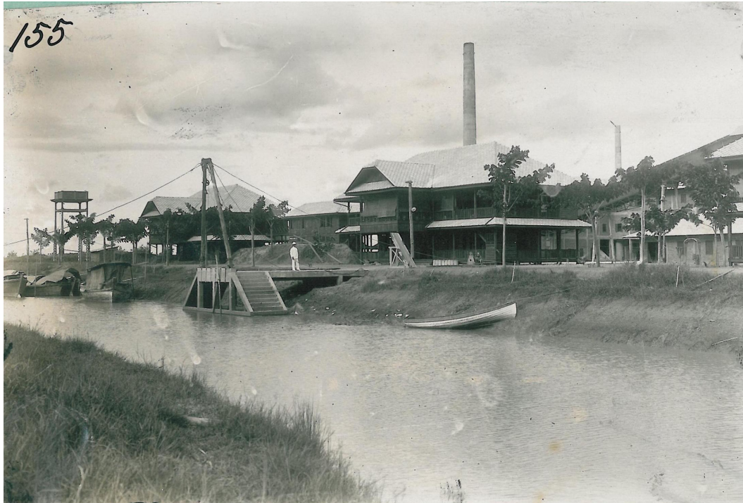
Living quarters for the Danish engineers and managers of the Siam Cement Co. plant in Bangsue in 1916. The production facilities can be glimpsed in the background.
