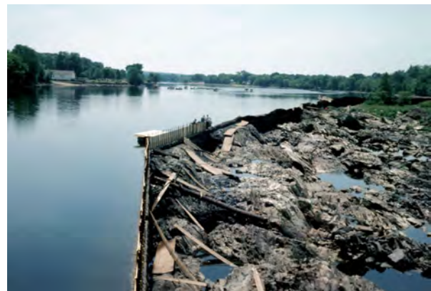
The flashboards on Pawtucket Dam being repaired or replaced in 1975.
