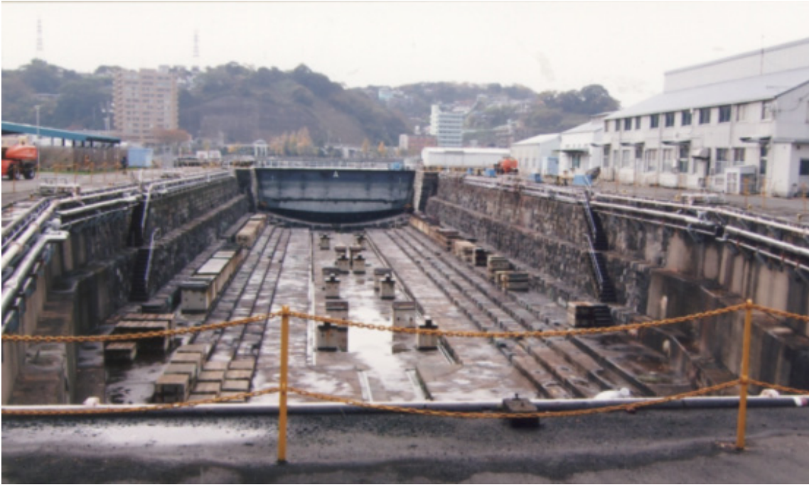
Yokosuka No.1 Dry dock: The first dry dock built with stone in Japan (1871)
