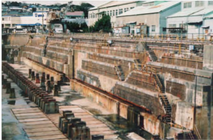
Fig. 2 - Uraga No.1 dry dock built with soil bricks (1899)
