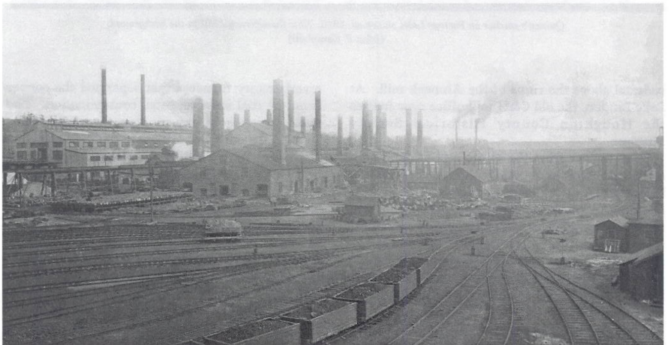
Myriad stacks, most rising from reverberatory furnaces, extend skyward at the C and H smelter in Hubbell. (MTU Archives and Copper Country Historical Collections)
