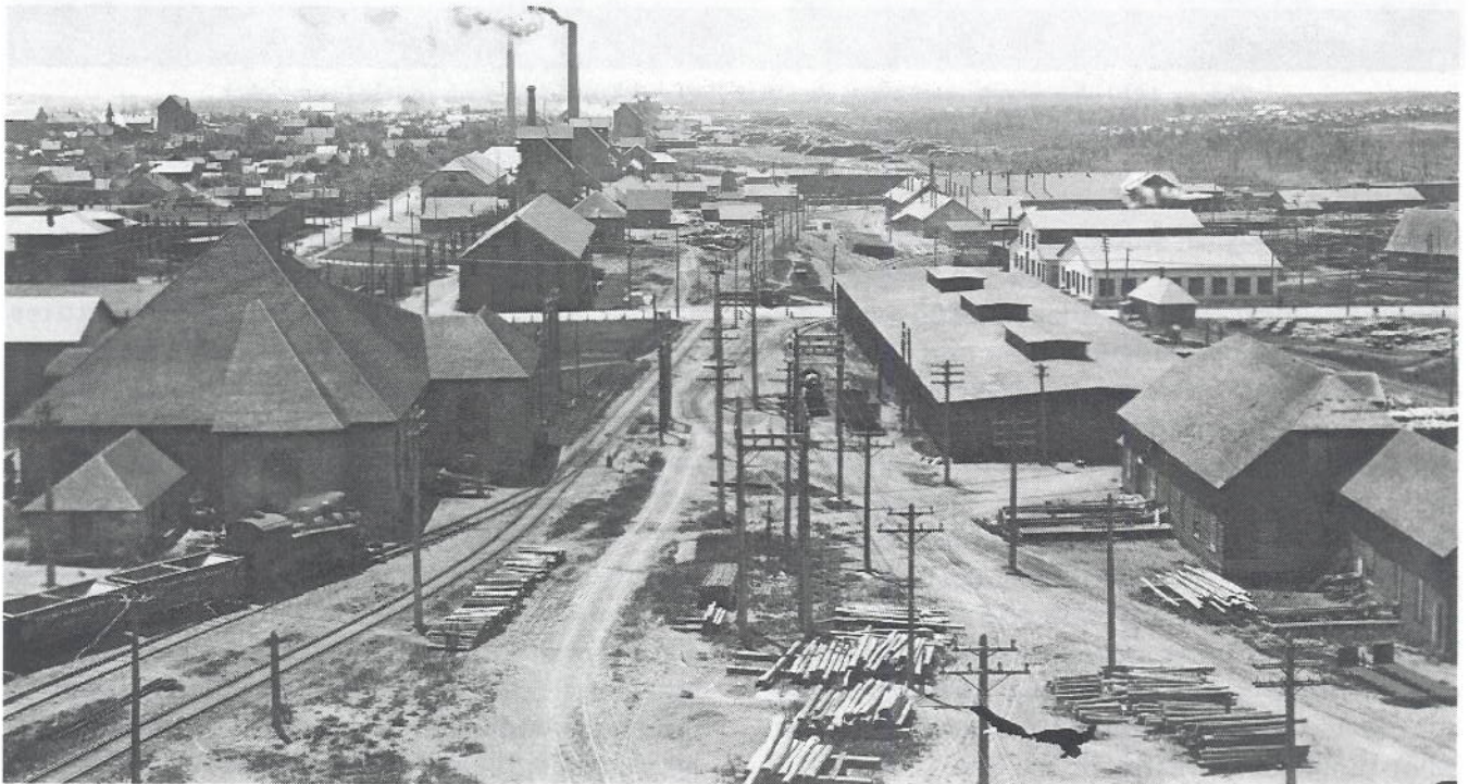
This ca. 1910 view of the C&H mine looks southwestward along the line of shafts that then paralleled Mine Street. Red Jacket Road passes from left to right at the center of this scene. (MTU Archives and Copper Country Historical Collections)
