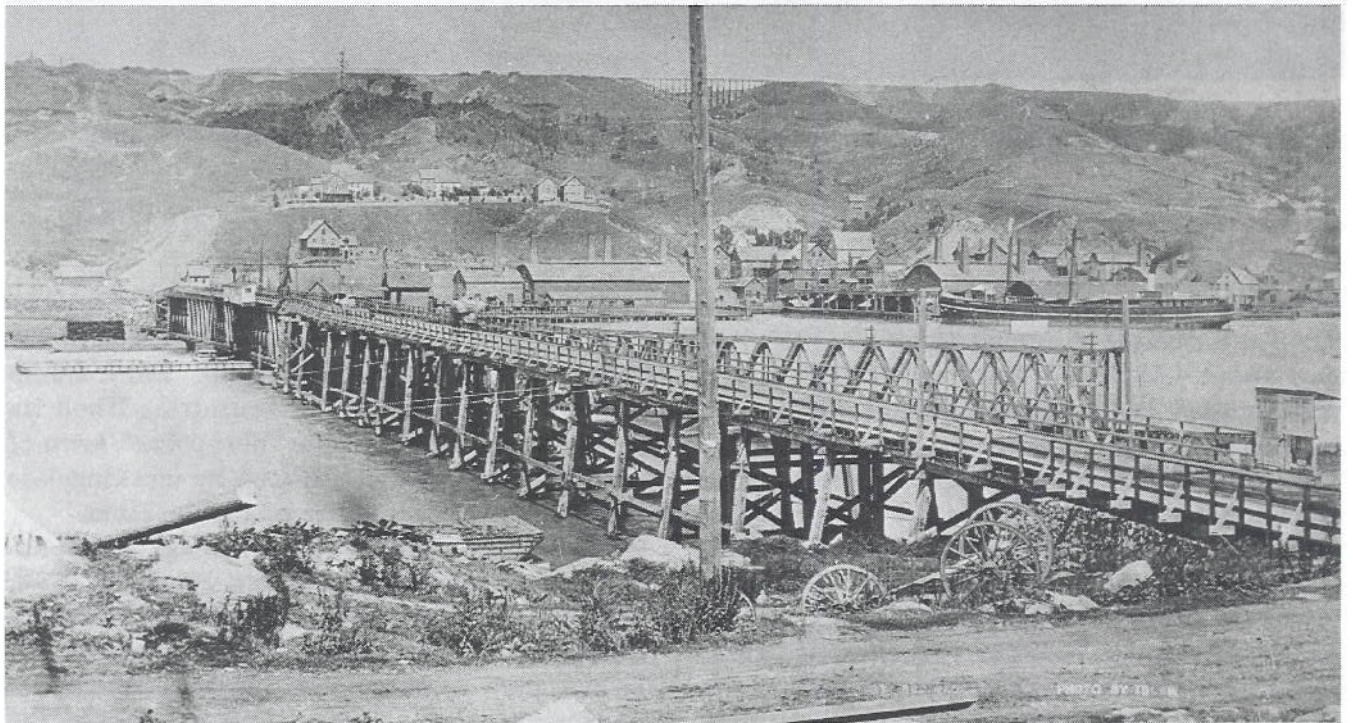
A wooden bridge, with a swing section to accommodate ships, opened between Houghton and Hancock in 1876. On the Hancock-Ripley side of the Portage, a large lake boat is shown docked at the Detroit and Lake Superior smelter. The modern double-deck lift bridge over the Portage was completed in 1959. (MTU Archives and Copper Country Historical Collections)
