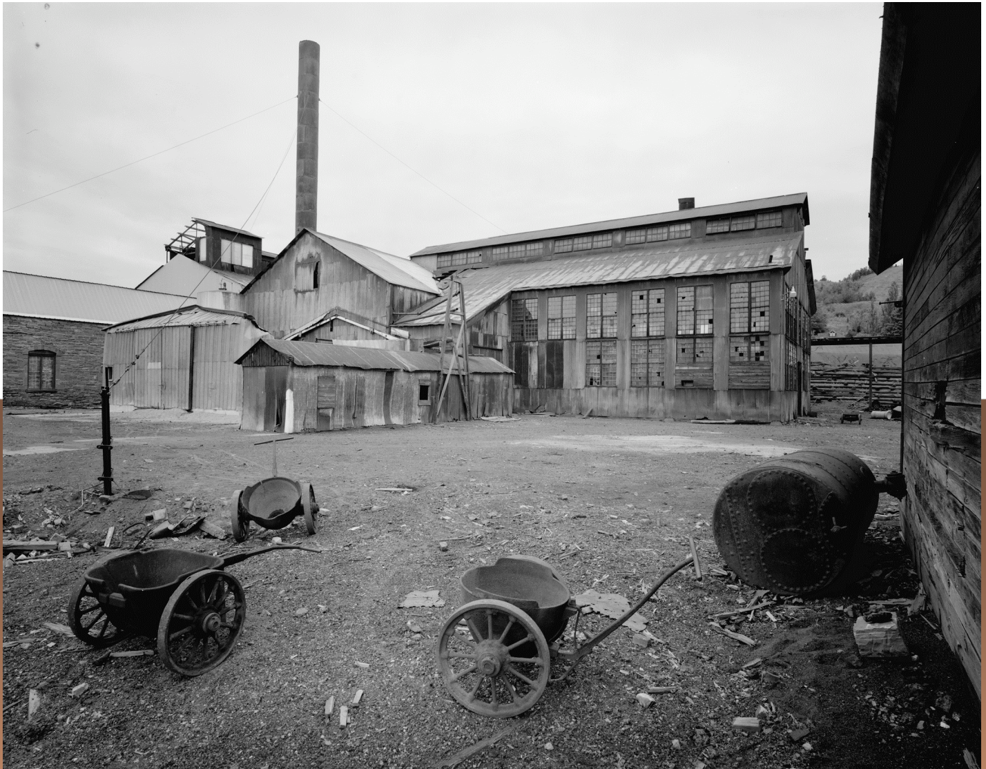
Quincy Smelter, Ripley, Michigan. Jet Lowe 1978
