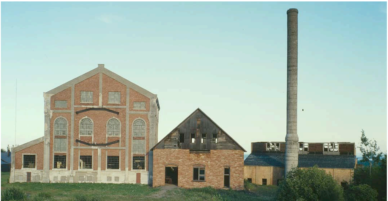
Mine buildings atop Quincy Hill. Jet Lowe.
