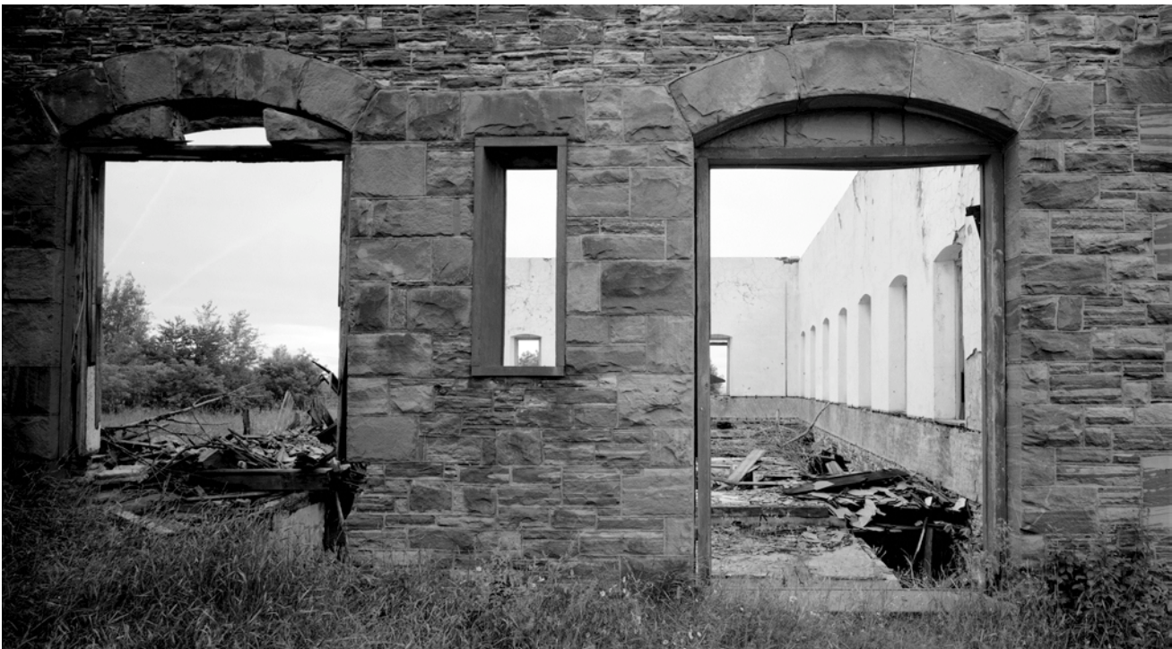
Ruins No. 7 Hoist House, built 1898-1900, Quincy Mine. Photographer: Jet Lowe.
