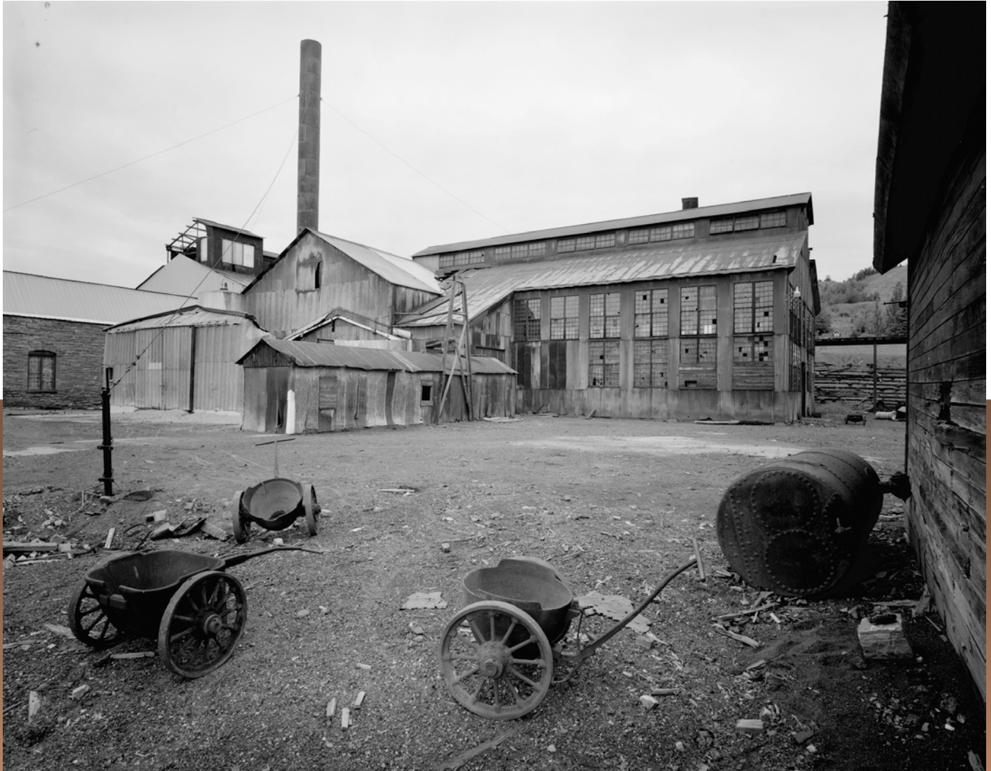
Quincy Smelter, Ripley, Michigan. Jet Lowe 1978
