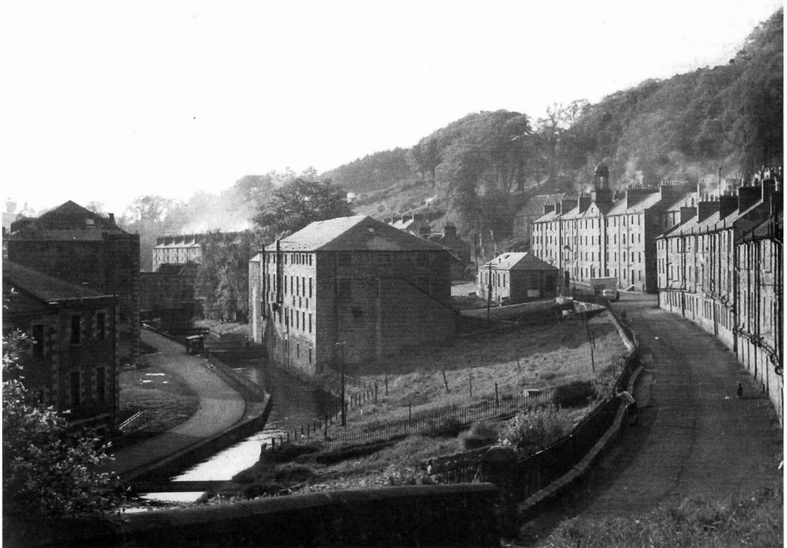
Figure 1.5 New Lanark (c. 1970), Robert Owen's model industrial settlement, is one of a group of industrial sites being submitted by the United Kingdom government for World Heritage designation. (Neil Cossons)
