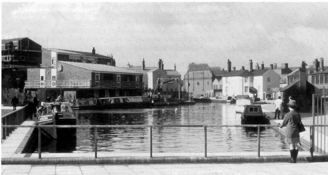
Figure 2.7 Brindley Walk, Birmingham. A successful redevelopment of an inner-city industrial site, shown here soon after its restoration in 1969. It is a basin formed by a branch off the Birmingham & Fazeley Canal built by James Brindley in the eighteenth century. (R A Buchanan)
