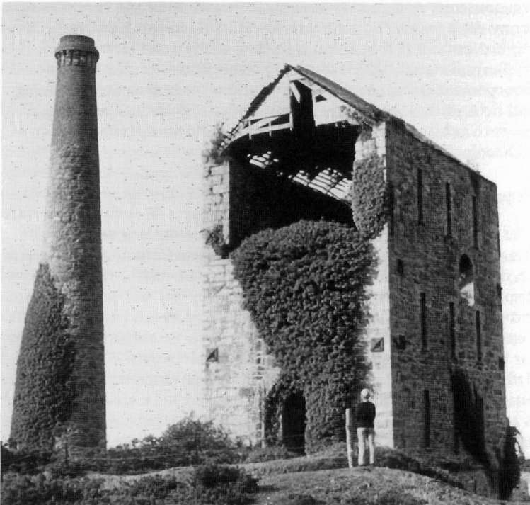
Figure 2.2 Cornish Engine House in ruins at Tregurtha Down, Penzance, in 1978. This building is very typical of west Cornwall, where many substantial monuments of the tin and copper mining industry survive. (R A Buchanan)
