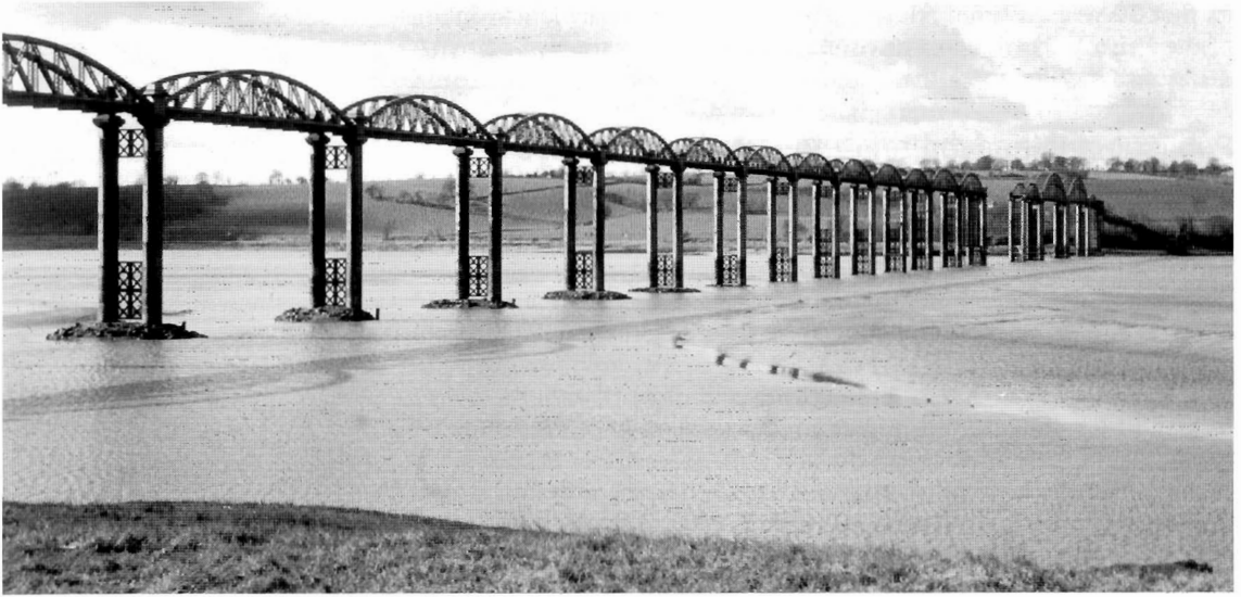
Figure 2.4 Severn Railway Bridge, Sharpness, seen here during a BIAS visit in 1968. The bridge had been closed to traffic since a barge had collided with a pier at the far end and demolished two spans. It was subsequently dismantled and sold in parts. (R A Buchanan)
