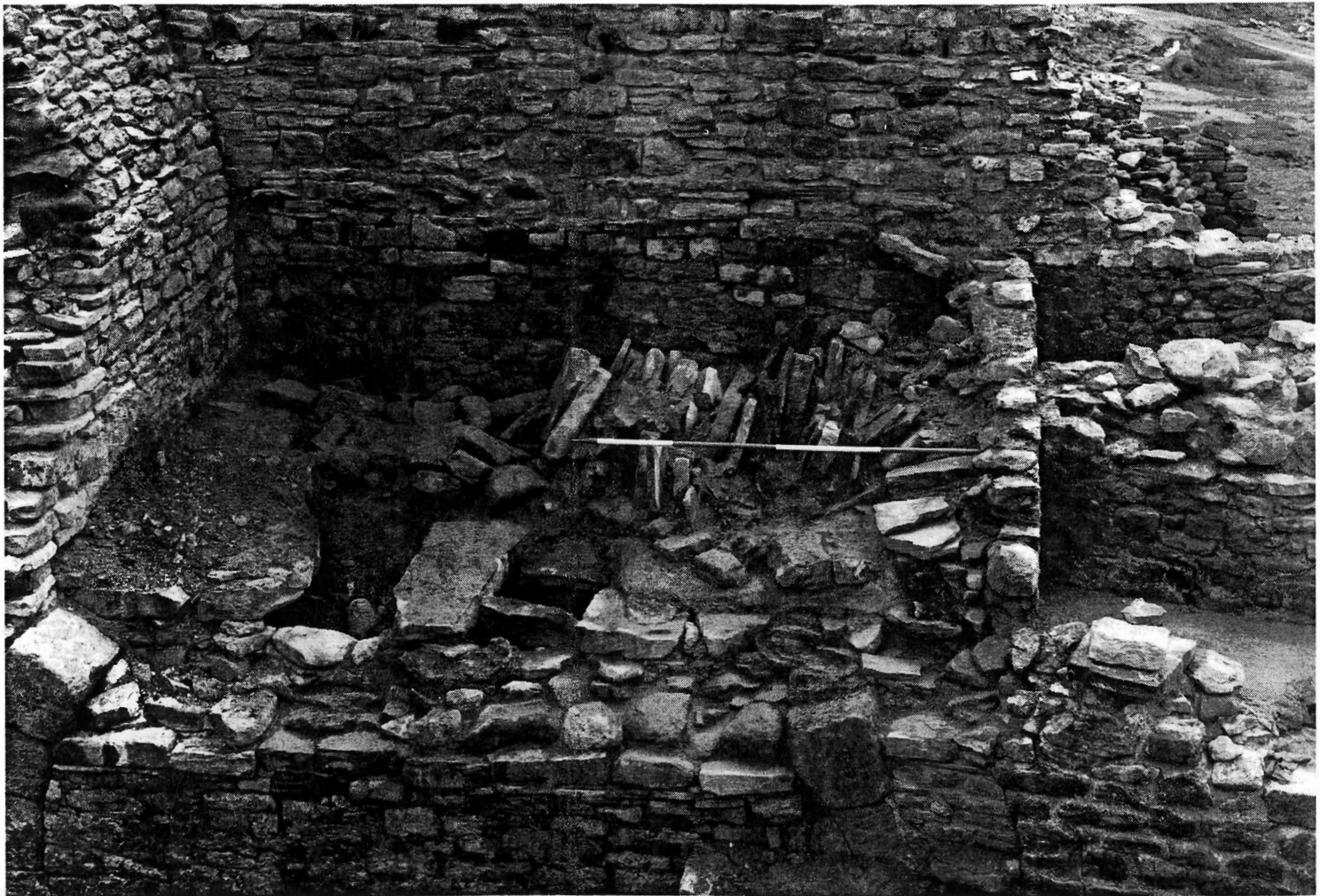
Plate 1 Old Gang Smeltnill: the rubble behind the scale is the collapsed face of the wall to its right, and cleaning has revealed a strapping beam within it (above the centre of the scale).
