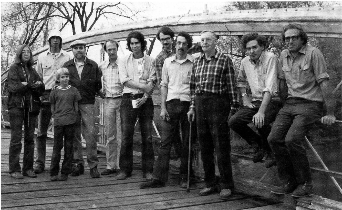
Figure 13. Montgomery C. Meigs original chapter, SIA (from the Washington, DC area), November 8, 1975, Keysville Road Bridge, over the Monocacy River near Keymar, Md. The bridge (c. 1875), a column, plate, and channel-type fabricated by the Wrought Iron Bridge Company of Canton, Ohio, was recorded with hopes that the effort would dissuade county engineers from replacing it; however, the bridge was destroyed shortly after recording. Members (left to right) are Sandra DeLony, Alan Nelson, Lars Sande, first SIA President Ted Sande, Eric DeLony, Donald Jackson, Phillip Speiss, Bob Hoke, Charles Looney, Peter Stott, and Robert Vogel. Photographer unknown.
