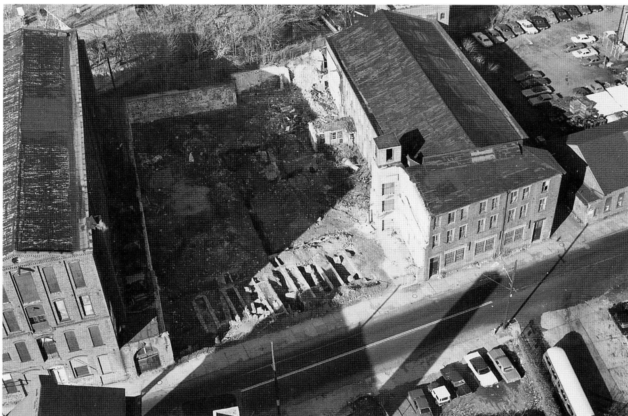
Figure 10. Great Falls-SUM Survey, summer 1974. Fortuitous circumstances allowed simultaneous above- and below-ground archeology in this project when a HAER team worked with industrial archaeologist Edward S. Rutsch, whose dirt-archeology team revealed the locomotive bays in a demolished portion of the former Grant Locomotive Shops in Paterson, N. J., and located head and tail races running along the tree line in this photograph. The combined skills of the two teams produced a documentation package that was unprecedented for the new, emerging field of industrial archeology. Jack Boucher, HABS/HAER photographer.
