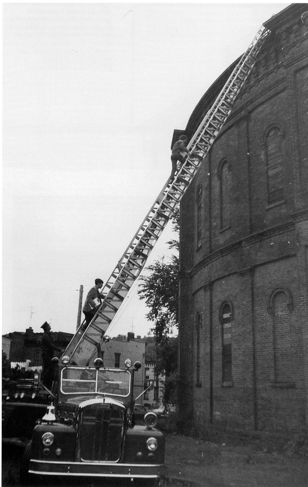
Figure 8. Troy, New York, fire department's hook-and-ladder truck. Used by David Bouse and Charles Parrott III in June 1969 while measuring cornice of Troy Gasholder house. Robert Vogel, Smithsonian Institution, photographer.
