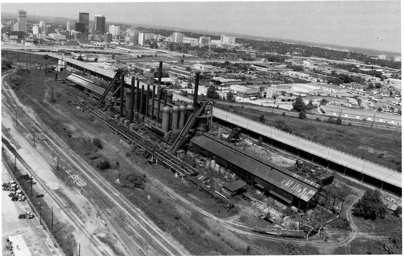
Figure 16. Context of Sloss Furnaces, Birmingham, Alabama. Though Birmingham, the cast-iron center of the world, is not yet officially designated a heritage area, its citizens saved the Sloss Furnaces in 1976, one of the first major industrial archeology preservation efforts in the south. Led by Marjorie Longnecker White, president of the Birmingham Historical Society, people are working to carve out the "Birmingham District," a five-county heritage area that will save and interpret the history. Photography by Garrison's Flying Photo, photographer unknown.
