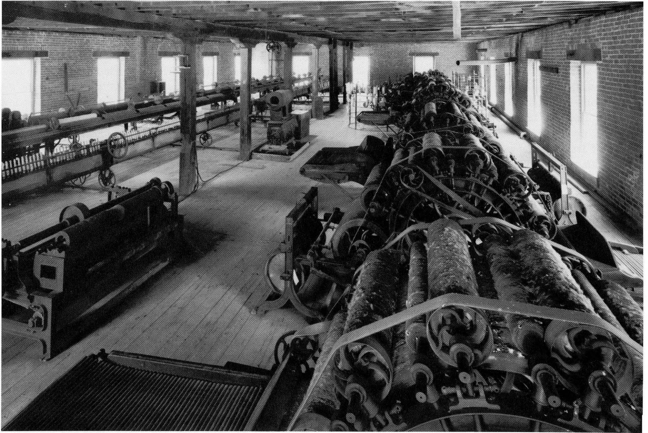
Figure 9. Carding and spinning room. Note joisted floor above.
