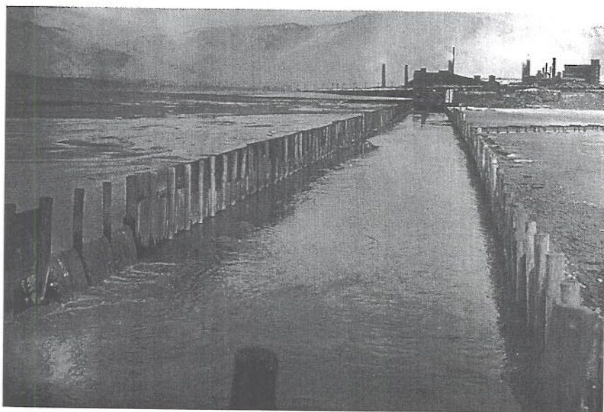
Figure 3. This photo, presented as evidence in 1905 in Magone v. Colorado Smelting and Mining Company, et al , shows an open "culvert" carrying Silver Bow Creek through the tailings impoundments at the Butte Reduction Works at Butte, Montana. Water flowing into the culvert on the left is the overflow from an impoundment where solid tailings have settled after having been discharged from the concentrator at the smelter, visible in the background. Such a technology for managing industrial wastes would not normally have attracted the attention of a photographer, had it not been for the trial. Photo courtesy of the National Archives, Seattle Branch.
