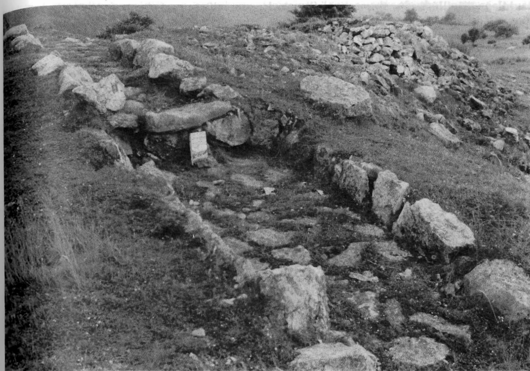
FIGURE 1. Different kinds of buddles in use in 19th-century and early 20th-century mineral dressing. Opposite, above: Concrete faced convex centre head buddle constructed at West Basset, Cornwall. c. 1874.
