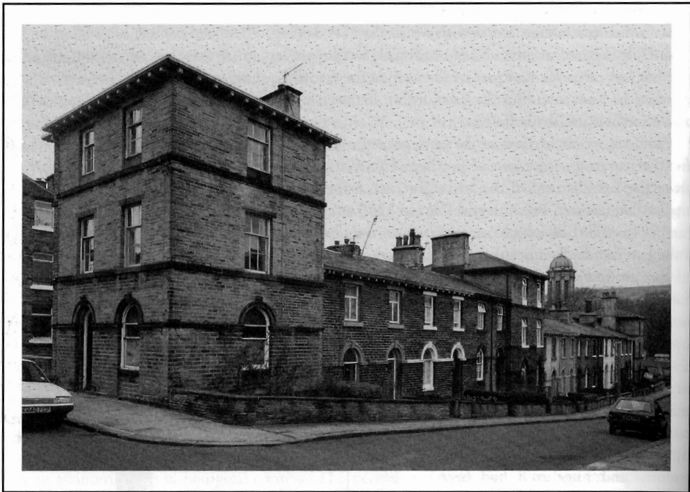
Plate 2 Workers' housing in William Henry Street, Saltaire, West Yorkshire, built 1854. The varied façades mirror the social hierarchy within the mill. The tall end blocks were intended for boarding houses, while the elaborate stone lintels and front gardens of the terraced houses reflect the status of the overlookers who occupied them. The cupola of Sir Titus Salt's elaborate Congregational church can be seen in the distance.
