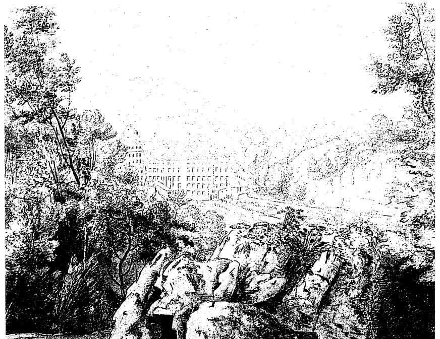
Fig 22 Cromford Mill, Derbyshire (below). Richard Arkwright built the first water-powered cotton mill at Cromford in 1771. By 1790 it had become part of a group of multi-storey spinning mills and warehouses. This view by William Day (1789) shows the rural setting for the cradle of Britain's cotton manufacturing industry where Arkwright's techniques of factory production were developed and copied throughout the world. Cromford Mill was acquired by the Arkwright Society in 1979; with the help of English Heritage grants and with funding and sponsorship from many sources, the site is gradually being restored for a variety of uses with interpretation for visitors. (Print reproduced by courtesy of Derby Museums and Art Gallery)
