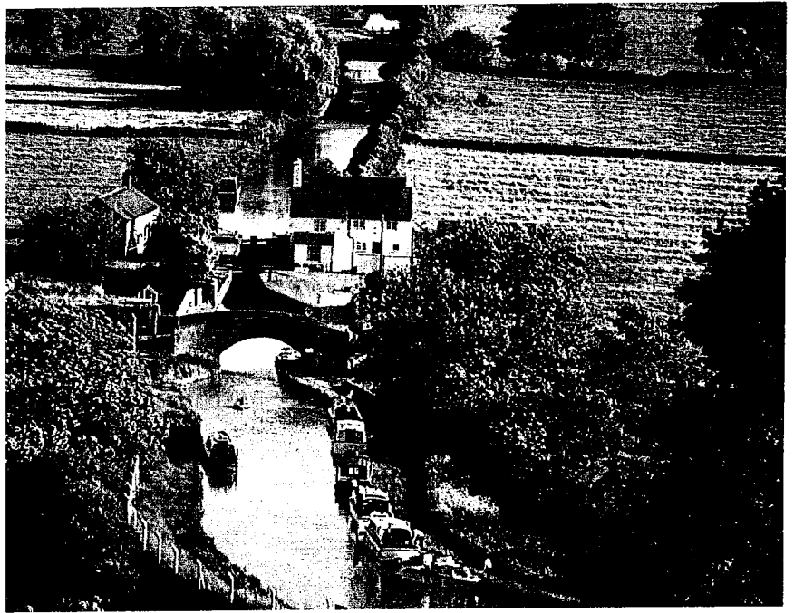
Fig 10 Oxford Canal, Napton, Warwickshire. Construction of the Oxford Canal, begun in 1769 under the distinguished engineer James Brindley, was typical of the early so-called 'contour canals'. By following the contours of the land, the costly engineering of tunnels and aqueducts was avoided. Typical among rural canals in the Midlands, this view of the Oxford Canal at Napton includes examples of the brick structures which contribute to the distinctive architectural character of inland waterways. English Heritage has funded jointly with British Waterways an Architectural Heritage Survey providing information for a computerised database to help with conservation and management of historic waterway structures. (Photograph reproduced by courtesy of British Waterways)
