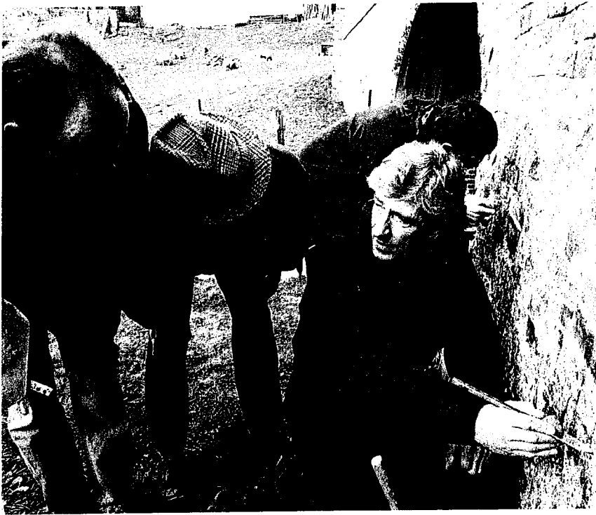
Fig 21 Braunston, Northamptonshire (left). English Heritage is providing conservation training for British Waterways staff. On this canal accommodation bridge at Braunston, Northamptonshire, techniques of cutting out defective mortar and careful repointing are demonstrated on site by specialists from the English Heritage Training Centre at Fort Brockhurst. (Photograph courtesy of British Waterways)
