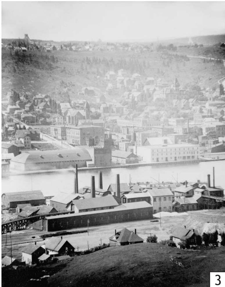
(ABOVE) 2. Quincy Smelting Works south side overview, as seen from Houghton c. 1910 (neg. 01316, HAER MI-2-174, courtesy of MTU Copper Country Archives)
