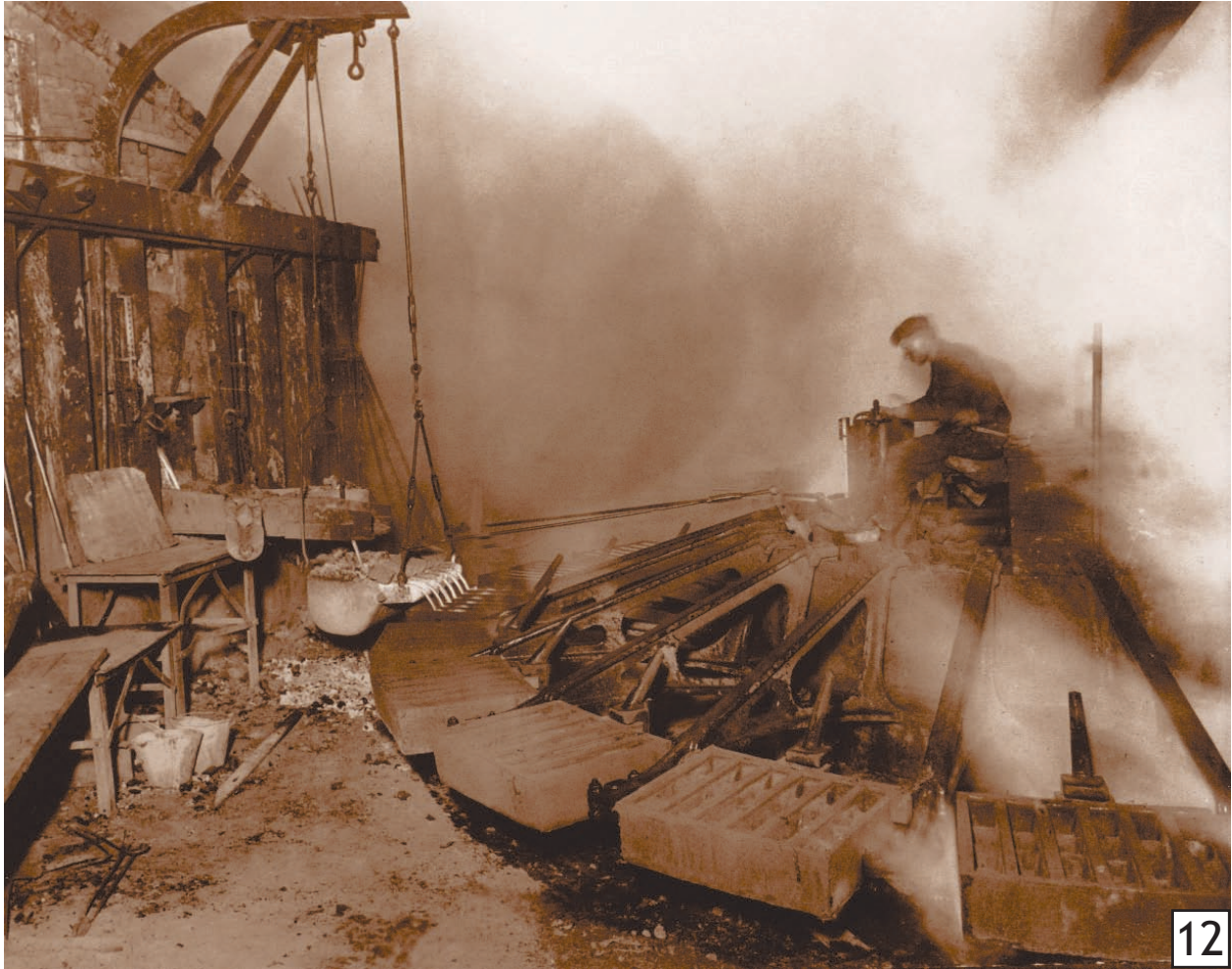
12. Worker operating a Walker Casting Machine at the Calumet & Hecla smelter, Lake Linden, MI c.1900. ( collection of Views of the Past, Marquette, MI )
