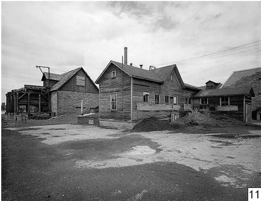
11. Left: Charcoal house, center: assay office. (HAER MI-2-210 photo by Jet Lowe, 1978)
