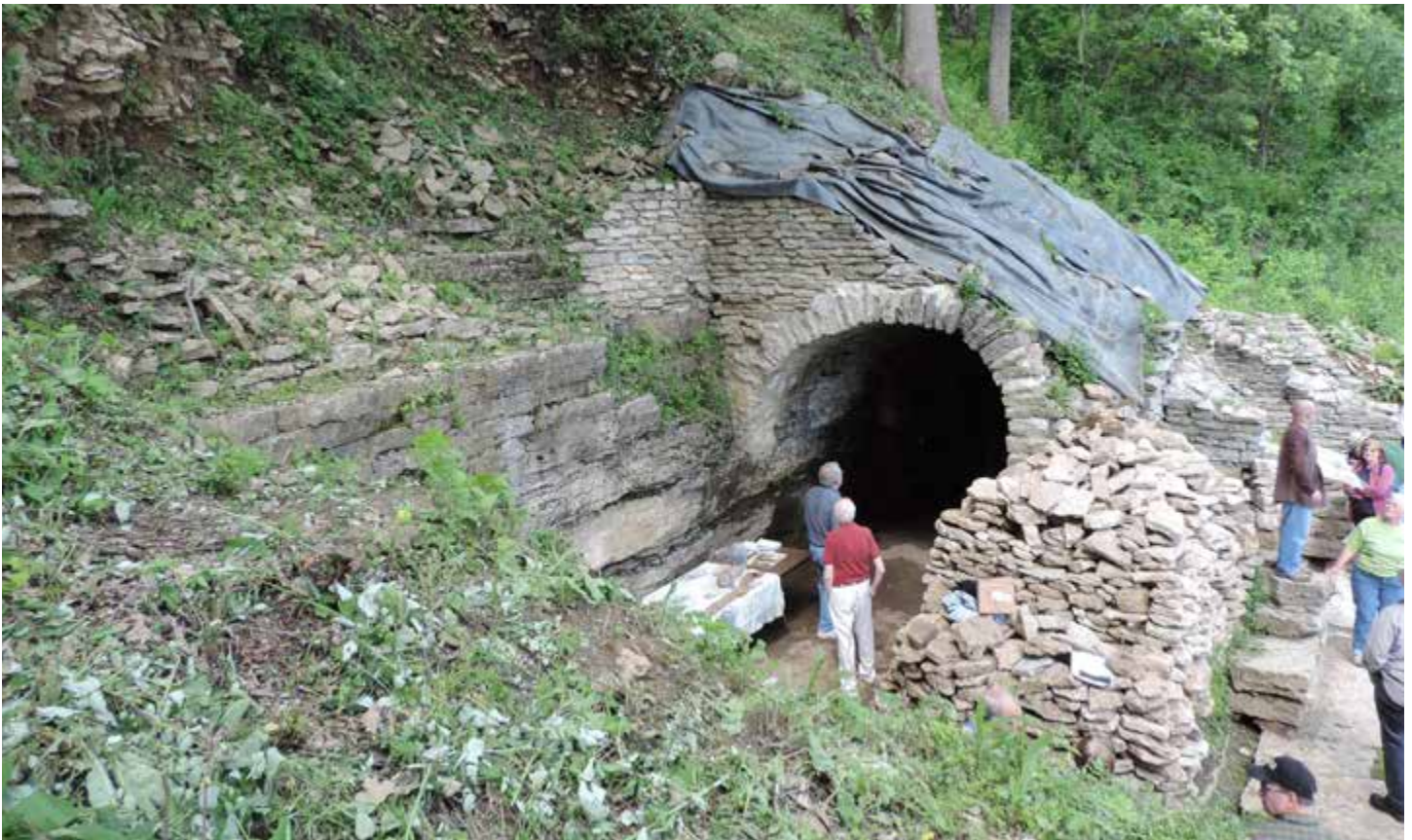
Excavation of British Hollow Lead Smelter, Potosi, Wisconsin.
