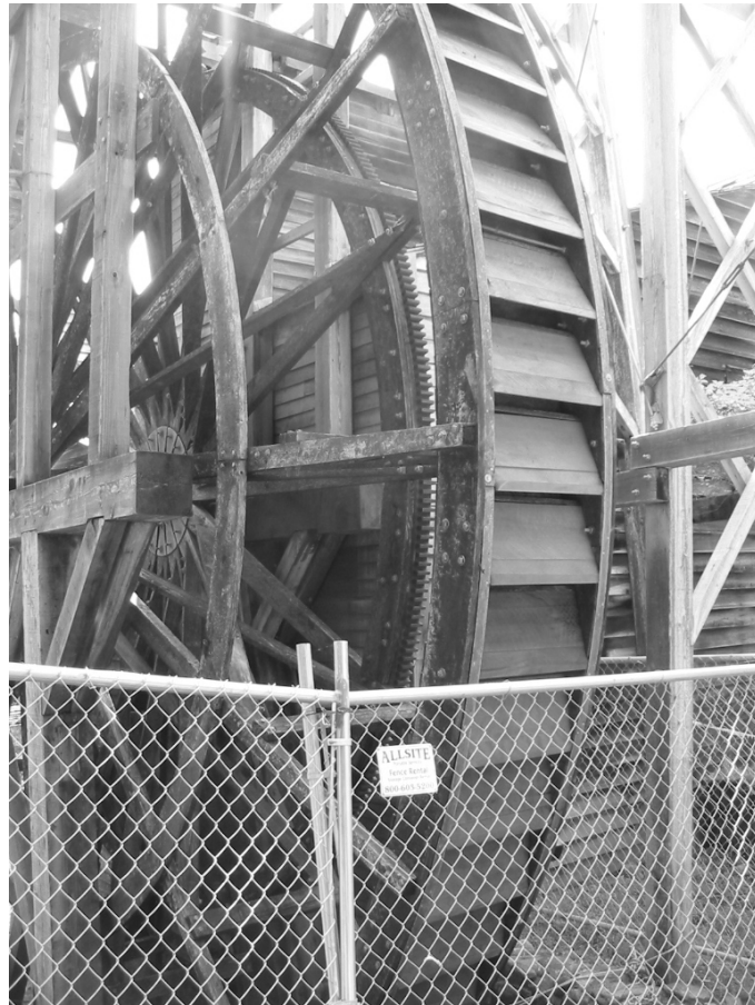
Overshot Wheel at Bale Mill. Note the main drive gear inside the ring of buckets.
