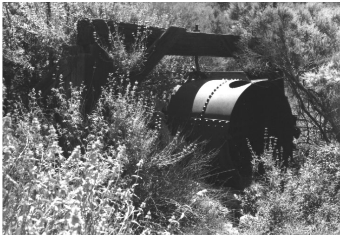
Boiler at Houston and Cohn
