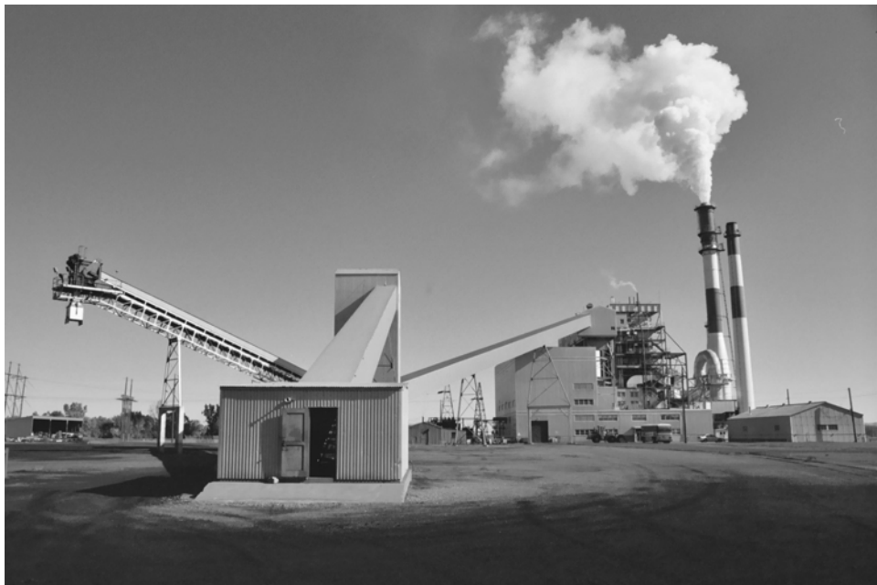
Lewis and Clark Power Station
