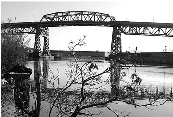
Kosciuszko Bridge over Newtown Creek.
