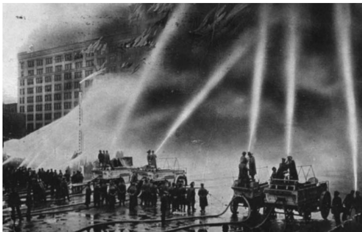
Based on comparison to images in Engineering News, this is actually the Oct. 22, 1908 test of the High Pressure Fire System at West and 12th Sts. The flames are painted in.
