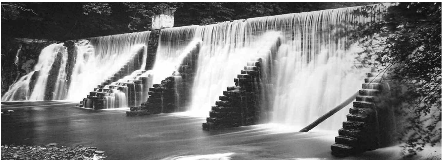
Lake Solitude Dam, High Bridge, NJ.
