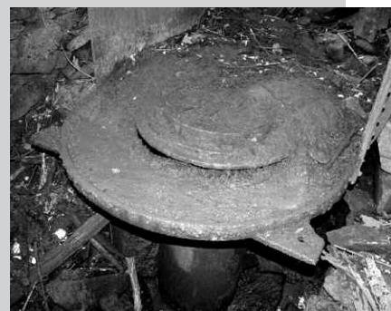
ABOVE: The cast iron top of the turbine housing at the Smith-Connet Grist Mill site has been broken, likely in the removal of the rotors in a scrap drive. The housing held a pair of inline turbines. The single penstock is visible in the lower left of the top photo.
