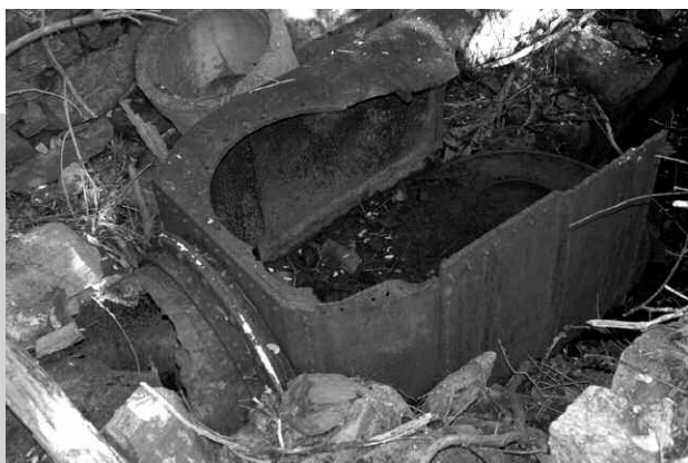
ABOVE: The cast iron top of the turbine housing at the Smith-Connet Grist Mill site has been broken, likely in the removal of the rotors in a scrap drive. The housing held a pair of inline turbines. The single penstock is visible in the lower left of the top photo.
