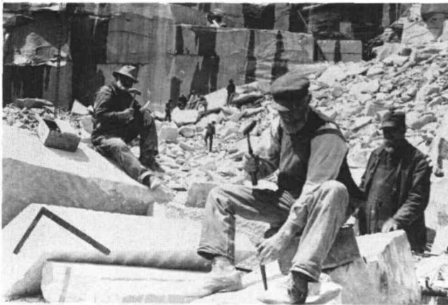
Figure 10. “Drilling Preparatory to Splitting, Concord, N.H.,” from a stereograph by the Keystone View Company, Meadville, Pennsylvania, c1910. According to a 1907 study by Halbert P. Gillette—Rock Excavation—“a good workman can drill and plug 80 holes in 8 hours.” The same study showed that “each man drilled each hole (9/8-in. diam. × 2½ ins. deep) in a trifle less than 5 mins., by striking about 200 blows. . . . Blocks 30 in. long, with four plug holes, were drilled and split . . . in 24 mins. on the average.” Courtesy of the New Hampshire Historical Society, F1168.
