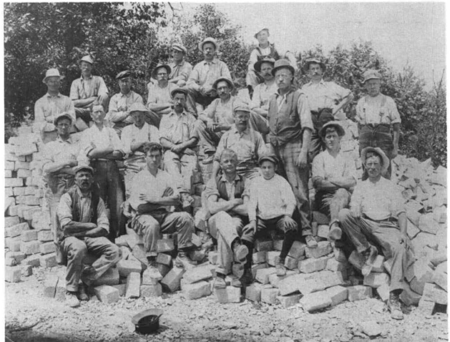
Figure 17. Pavement stonecutters, probably 1913. Paving blocks were quarried from the waste that remained after splitting building stone. By the end of the 19th century, New England was producing 60 million paving blocks annually. On the average a paving cutter could produce 100 stones per day. Granite manufacturer Ola Anderson, who lost his right arm in a quarry accident, appears here to the right of center wearing a bowler hat. Information courtesy of Reino Elgland and William P. Jones; photograph courtesy of New Hampshire Historical Society; gift of Thelma Colgan, F4209.
