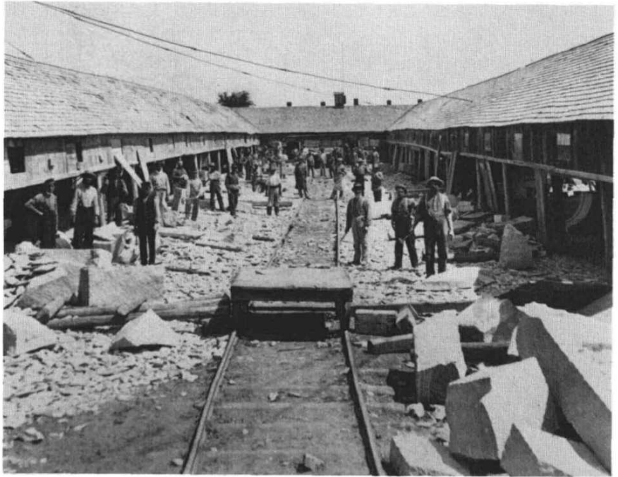
Figure 12. "Concord Granite Co. Looking North between the Sheds," from a stereograph by Howard A. Kimball, probably 1880s. By the turn of the century, Concord had 44 stonecutting yards where rough granite from the quarries was finished to serve a variety of purposes. The largest of these cutting plants employed 150 men and boasted 900 feet of sheds. Workers tended to specialize, whether in lettering, molding, carving, or plain work. Railroad sidings connected cutting yards to main lines. Courtesy of the New Hampshire Historical Society, F4207.
