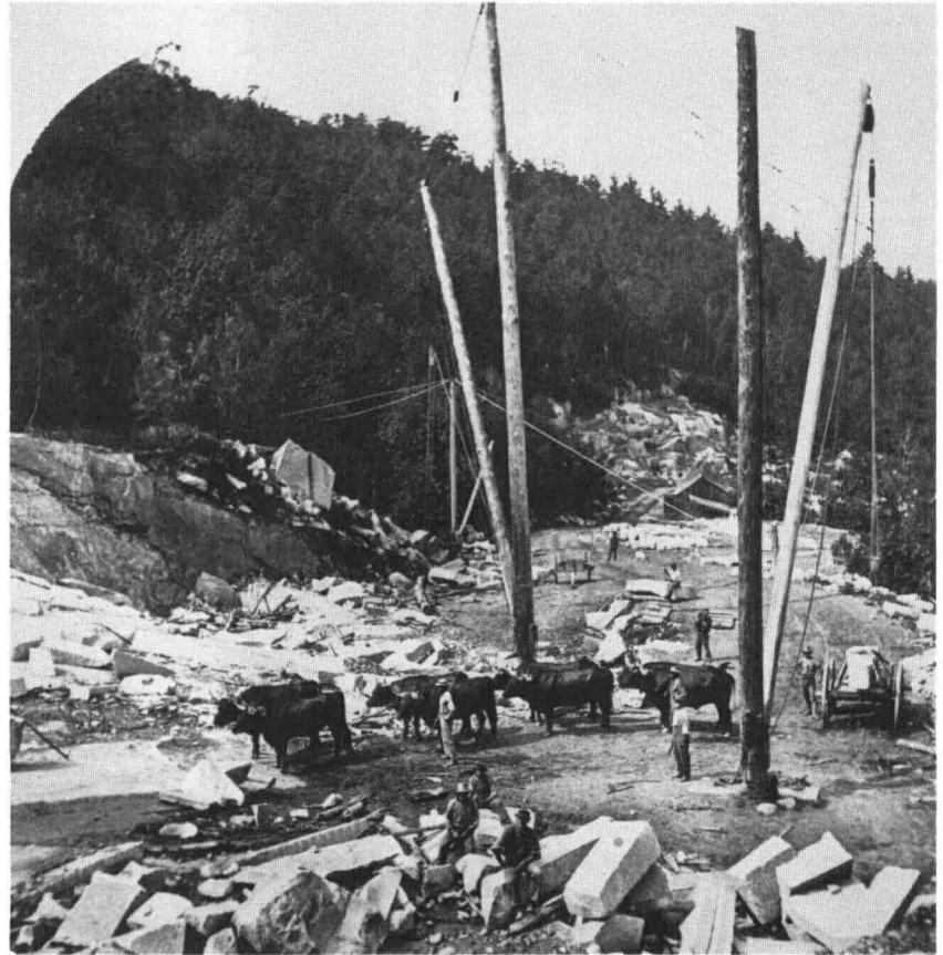
Figure 4. Four yoke of oxen in an unidentified Concord granite quarry, from a stereograph by Howard A. Kimball, c1870. Quarriers preferred oxen because of their calm temperament; they were used with derricks and wagons to hoist and transport granite. Sometimes, however, it was necessary to recruit as many as 40 yoke of oxen from nearby farmers to pull an especially heavy load. Courtesy of the New Hampshire Historical Society, N284.
