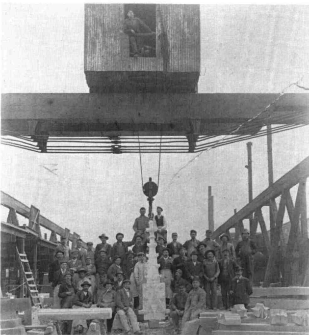
Figure 19. A traveling crane at the Swenson stonecutting sheds, photographed by the T. M. Knight View Co. of St. Louis, Missouri, c1910. Workers gather while a postcard photographer documents the completion of an ornamental crocket, probably for a church spire. Until recently, the Swensons specialized in building stone, the First Church of Christ Scientist in Boston and the Waldorf Astoria Hotel in New York being among their first major contracts. Courtesy of the New Hampshire Historical Society; gift of Judith F. Mason, F4205.
