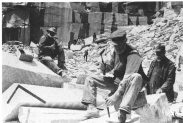
Figure 10. “Drilling Preparatory to Splitting, Concord, N.H.,” from a stereograph by the Keystone View Company, Meadville, Pennsylvania, c1910. According to a 1907 study by Halbert P. Gillette—Rock Excavation—“a good workman can drill and plug 80 holes in 8 hours.” The same study showed that “each man drilled each hole (3/8-in. diam. × 2½ ins. deep) in a trifle less than 5 mins., by striking about 200 blows. . . . Blocks 30 in. long, with four plug holes, were drilled and split . . . in 24 mins. on the average.” Courtesy of the New Hampshire Historical Society, F1168.
