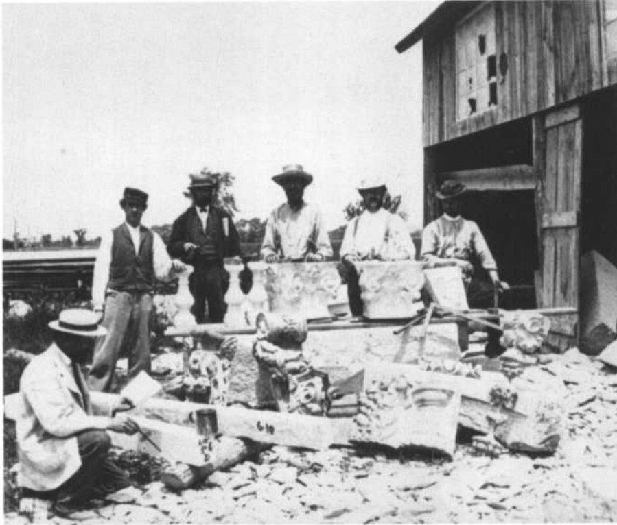
Figure 15. "Concord Granite Co., West Side of Carving Shed Looking North," from a stereograph by Howard A. Kimball, probably 1880s. "It may seem to an onlooker that it is a simple thing to chisel a line or bush hammer a stone, but care and skill are necessary from the time the stone is placed on [blocks] until it has passed inspection . . . and the paint mark, with the letter or figures of its position in the building, as shown on the plan, is placed on it by the person in charge"—Josiah B. Dyer, 1899. Courtesy of the New Hampshire Historical Society, N441.
