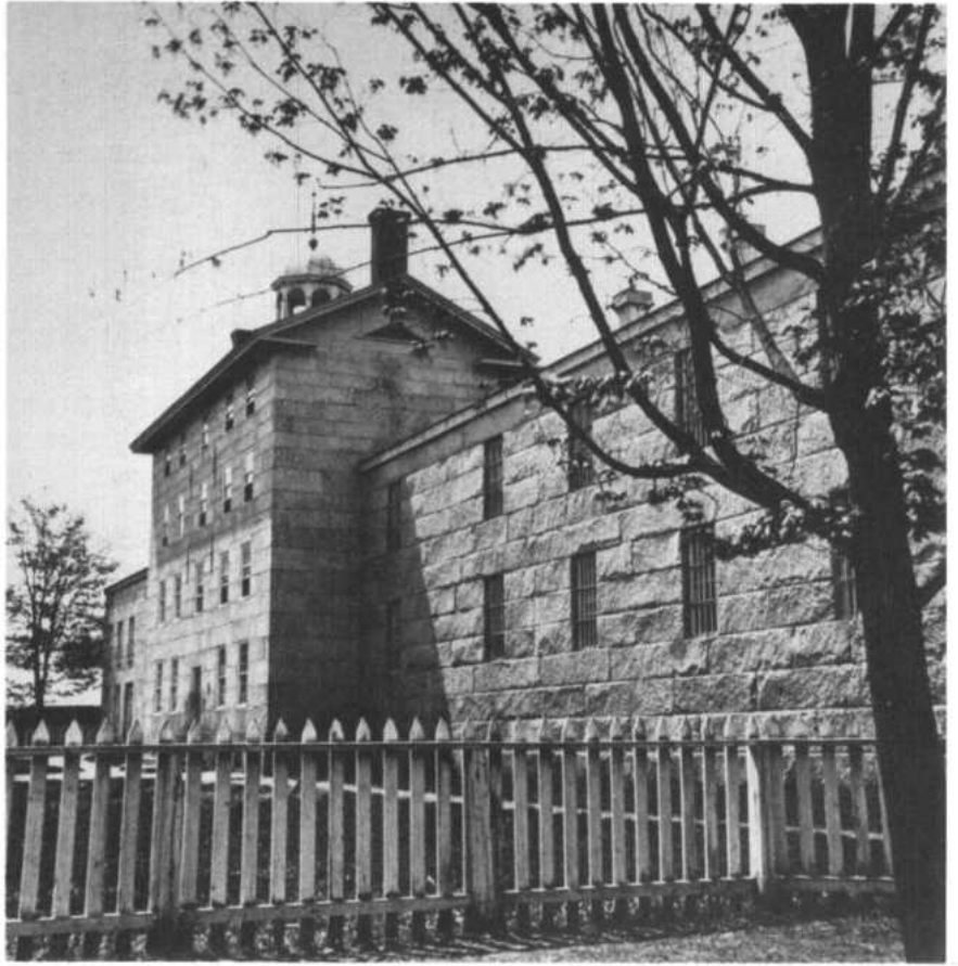
Figure 2. New Hampshire State Prison, Concord, constructed 1810, with additions dating from the early 1830s, from a stereograph by Howard A. Kimball, c1870. In many parts of New England, prisons were the first buildings constructed of split stone. Following Massachusetts's example, the Granite State supported its convicts by putting them to work cutting building stone for the nation's rapidly growing cities, thereby setting the stage for an important local industry. Courtesy of the New Hampshire Historical Society, N440.
