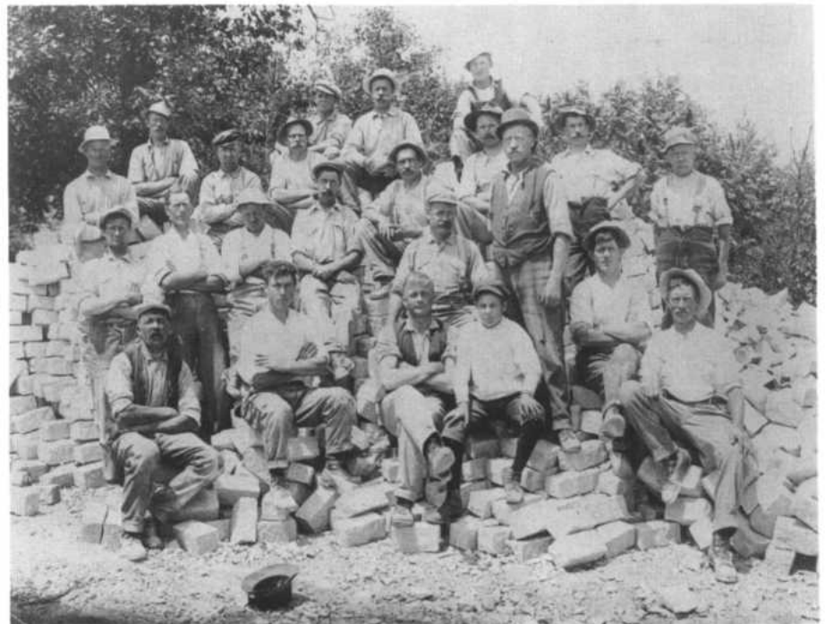
Figure 17. Pavement stonecutters, probably 1913. Paving blocks were quarried from the waste that remained after splitting building stone. By the end of the 19th century, New England was producing 60 million paving blocks annually. On the average a paving cutter could produce 100 stones per day. Granite manufacturer Ola Anderson, who lost his right arm in a quarry accident, appears here to the right of center wearing a bowler hat. Information courtesy of Reino Elgland and William P. Jones; photograph courtesy of New Hampshire Historical Society; gift of Thelma Colgan, F4209.
