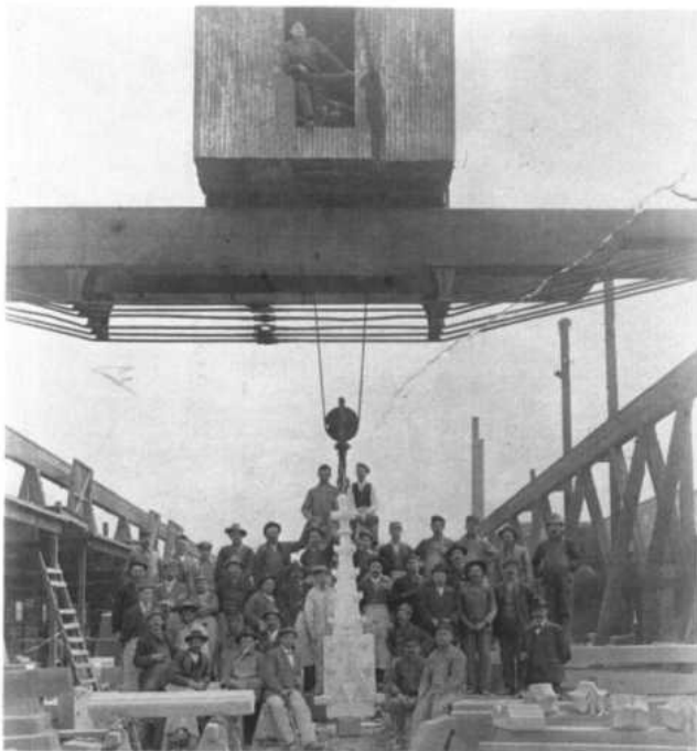
Figure 19. A traveling crane at the Swenson stonecutting sheds, photographed by the T. M. Knight View Co. of St. Louis, Missouri, c1910. Workers gather while a postcard photographer documents the completion of an ornamental crocket, probably for a church spire. Until recently, the Swensons specialized in building stone, the First Church of Christ Scientist in Boston and the Waldorf Astoria Hotel in New York being among their first major contracts. Courtesy of the New Hampshire Historical Society; gift of Judith F. Mason, F4205.
