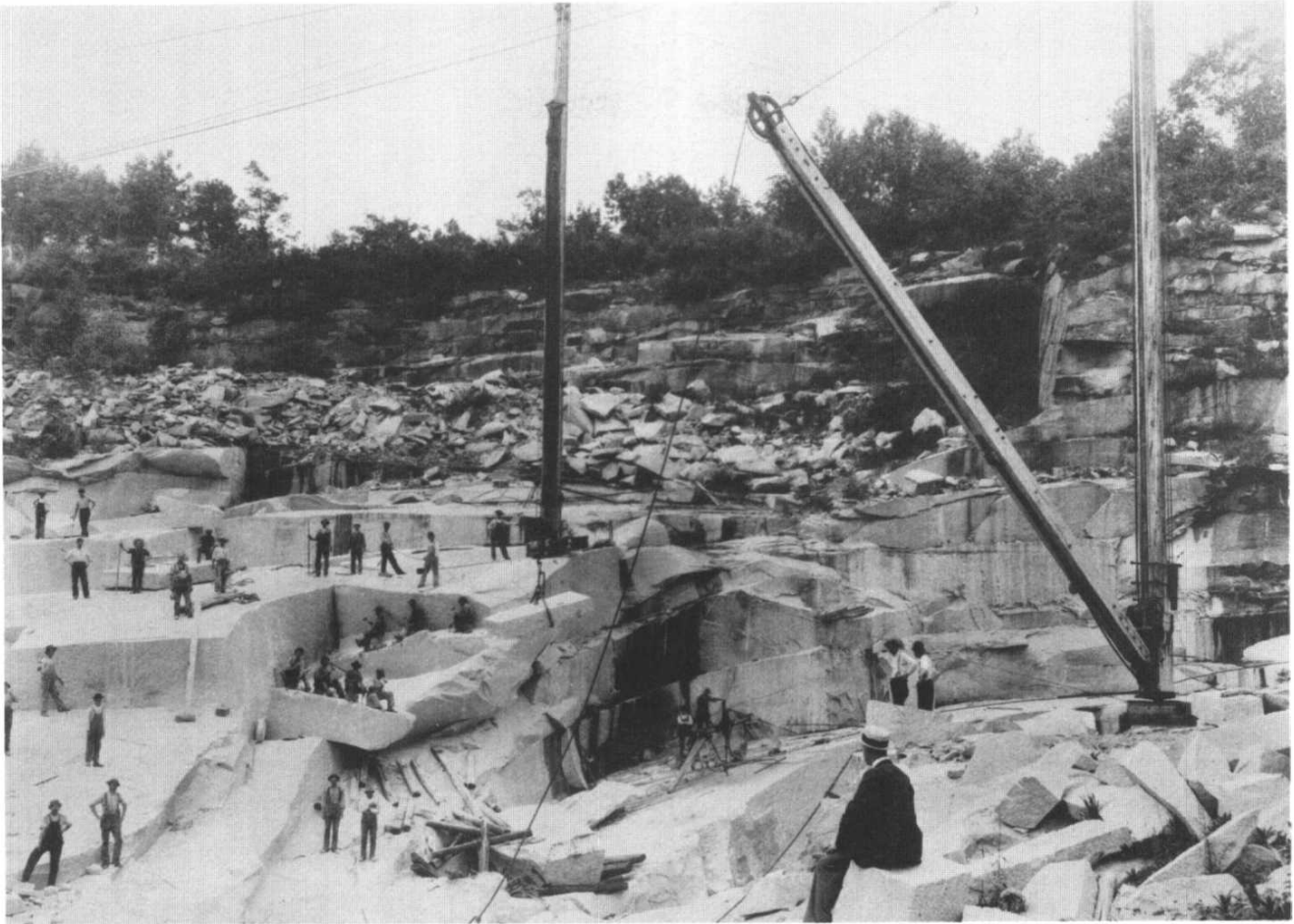
Figure 7. New England Granite Company Quarry No. 1 , published in Merrimack County Art Work , 1893. At left of center, two rows of quarriers coordinate their drilling, apparently oblivious to a large block of granite about to be lifted past them. This quarry was engaged at the time in supplying granite for the Library of Congress, the largest building project anywhere to that date. In 1896 the company employed 85 quarrymen, 154 granite cutters, 40 laborers, 2 machine men, and 12 tool sharpeners. Courtesy of the Concord Public Library, F4197.
