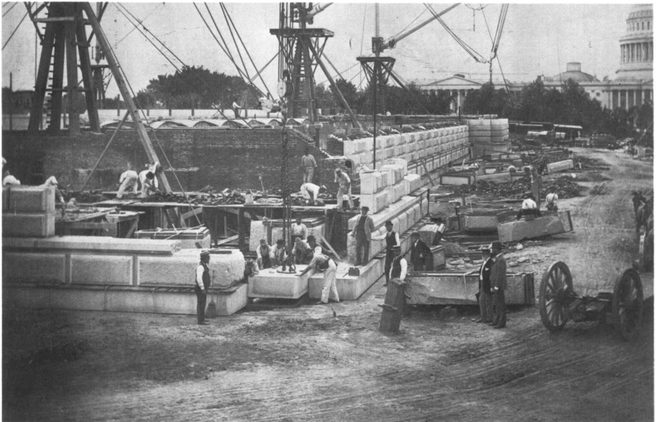
Figure 9. The laying of the cornerstone for the Library of Congress, Washington, D.C., August 28, 1890. To protect the corners and edges of the stone from being damaged in shipment, each block was boxed at the cutting yards. In this photograph, the wooden strips bound by iron hoops that have protected the granite are being removed so the blocks can be set in place. Courtesy of the Library of Congress.
