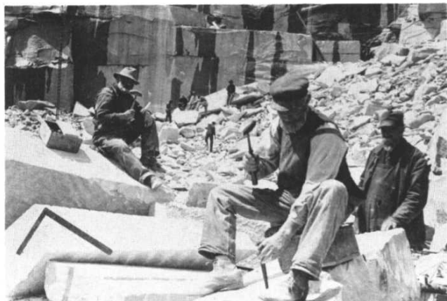
Figure 10. “Drilling Preparatory to Splitting, Concord, N.H.,” from a stereograph by the Keystone View Company, Meadville, Pennsylvania, c1910. According to a 1907 study by Halbert P. Gillette—Rock Excavation—“a good workman can drill and plug 80 holes in 8 hours.” The same study showed that “each man drilled each hole (3/8-in. diam. × 2½ ins. deep) in a trifle less than 5 mins., by striking about 200 blows. . . . Blocks 30 in. long, with four plug holes, were drilled and split . . . in 24 mins. on the average.” Courtesy of the New Hampshire Historical Society, F1168.
