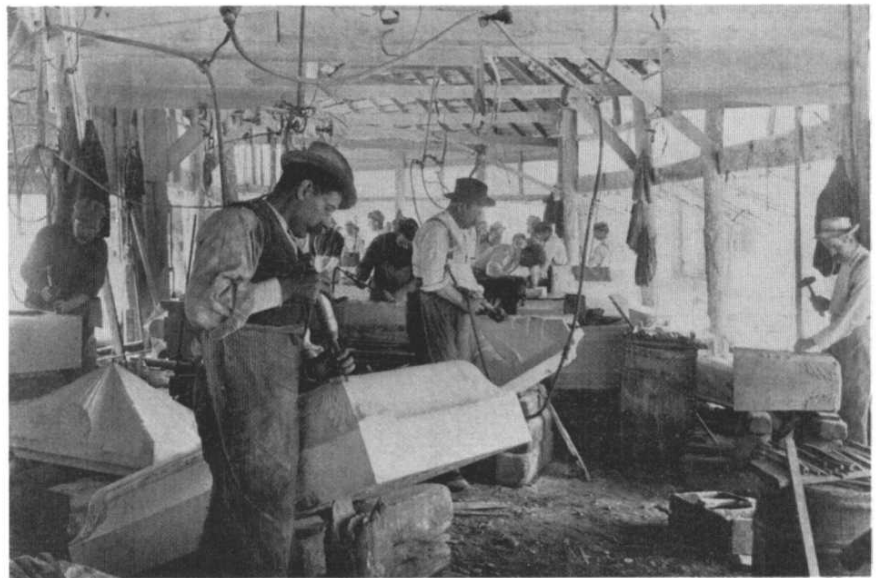
Figure 13. Interior view of William H. Perry's stone shed, Concord, from an advertisement published in Granite State Scenery, 1899. A native of Cornwall in England, Perry advertised his granite works as "equipped with all modern scientific appliances," including pneumatic tools and electric compressor motors. Even though the sides of the sheds were kept open as much as possible, granite dust filled the interior and was eventually identified as the cause of the chronic and pervasive lung disease silicosis. Courtesy of the New Hampshire Historical Society, F4206.
