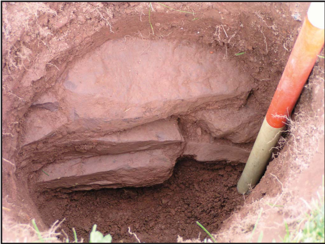
Plate 2. Hilltown Glasshouse [36Bu332]: View looking west of stone foundation observed in Shovel Test 12 located in the front yard of the Clauser property (Photographer: William B. Liebeknecht, June 2006) [HRI Neg.# 06033/D1:10].
