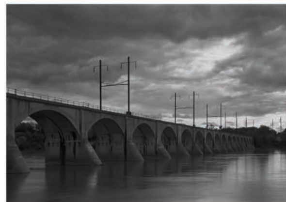
Cumberland Valley Bridge, Susquehanna River. Harrisburg, Pennsylvania
