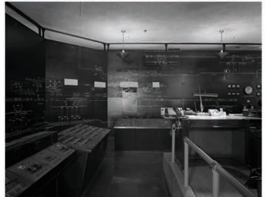
Power Dispatchers Office, Harrisburg Train Station Harrisburg, Pennsylvania
