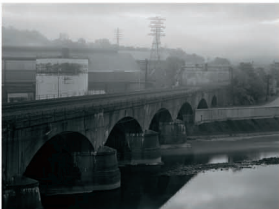
Conemaugh River Crossing and Cambria Works Johnstown, Pennsylvania
