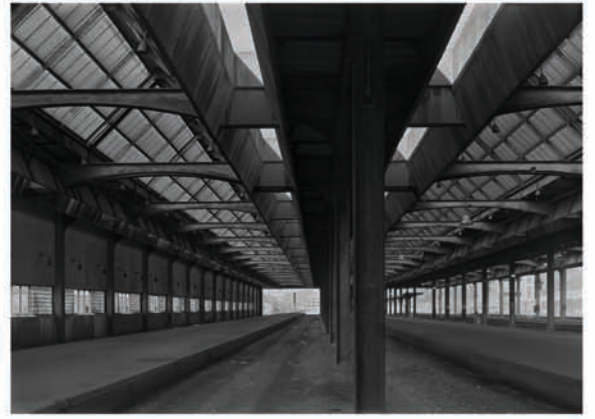
Train Shed looking East, Penn Station, Pittsburgh, Pennsylvania
