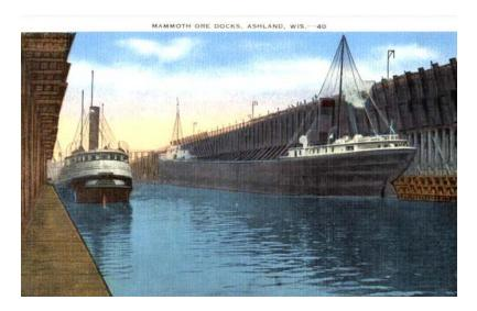
When originally built in 1916, the dock was 900 feet long and had a capacity of 52,000 tons of iron ore. In 1925, an expansion project doubled the ore dock's length to 1,800 feet, and increased its capacity to 110,000 tons. It was the largest active ore dock on the Great Lakes during that period of time.
