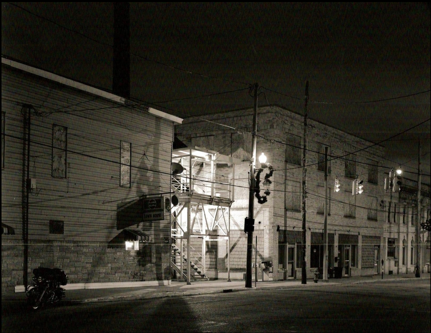
Worker entrance on Commercial Ave. leading to footbridge into mill. Mingo Junction, OH, Nov., 2012
