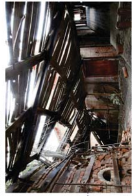
Framing system observed in the northwest end of kiln #4 shed. Wooden rafters are pulled to wooden runners. The wooden rafters sit on splayed iron angles that are anchored into metal post.
