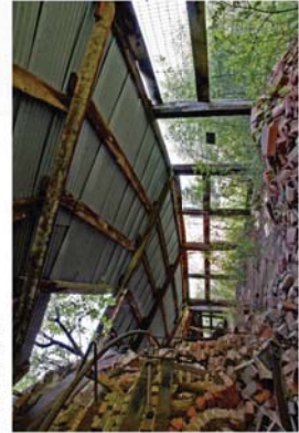
The only section of wood sheathing as a roofing material is found around the front entrance of kiln #4. This is thought to be the original roofing material.
