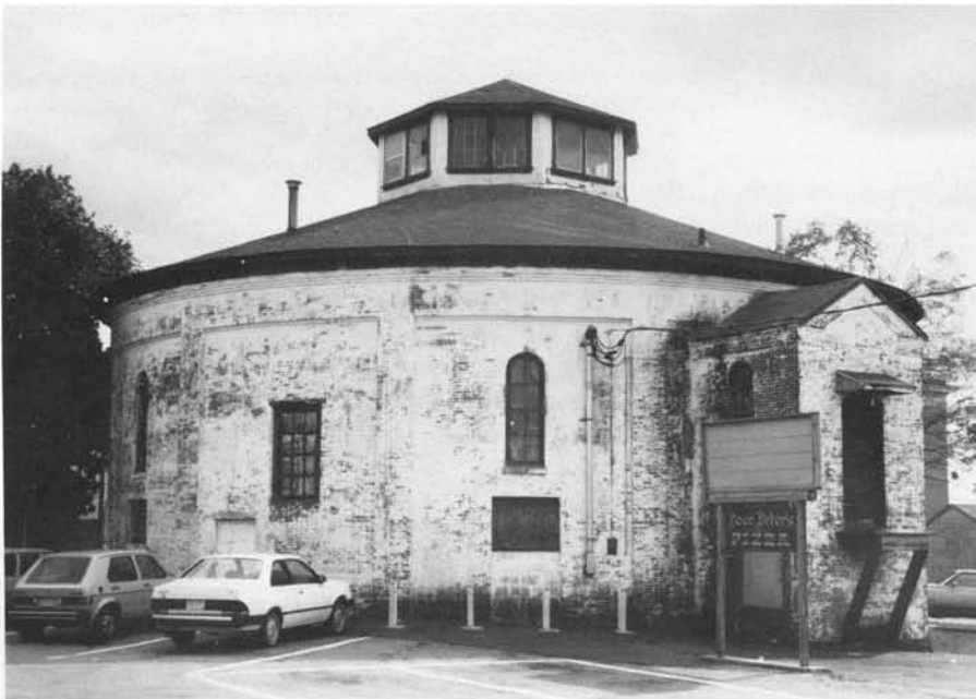
Figure 3. 1988 view of the East Street gasholder house in North Attleborough, Massachusetts. Photo by author.
