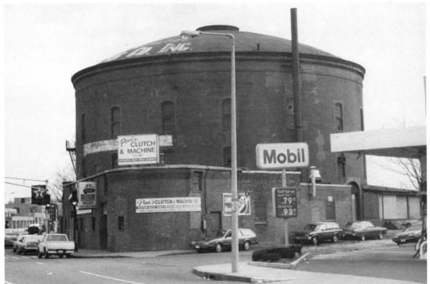
Figure 1. 1988 view of the gasholder in Roxbury, Massachusetts. Photo by author.
