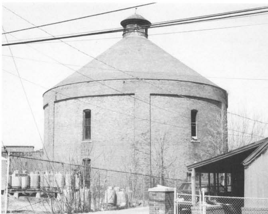
Figure 7. Gasholder in Biddeford, Maine, as viewed in 1988. Photo by author.
