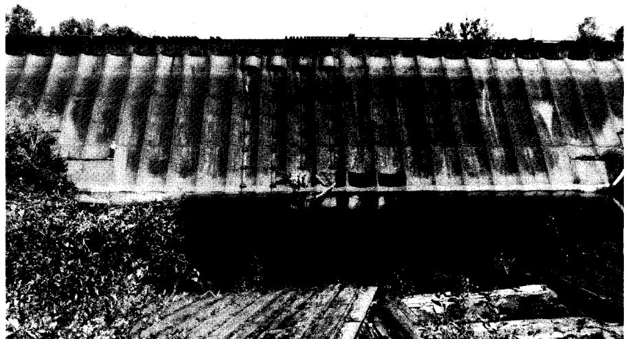
Figure 10. Water face of Redridge steel dam, 1988. View from the south taken from remnants of 1894 timber crib dam (foreground). Note sections of steel plate removed just above waterline (center of photo). These were cut out in 1979 to reduce water load on the dam. The railroad trestle which shares the concrete foundation of the dam is visible above the dam. Photo by Author.
