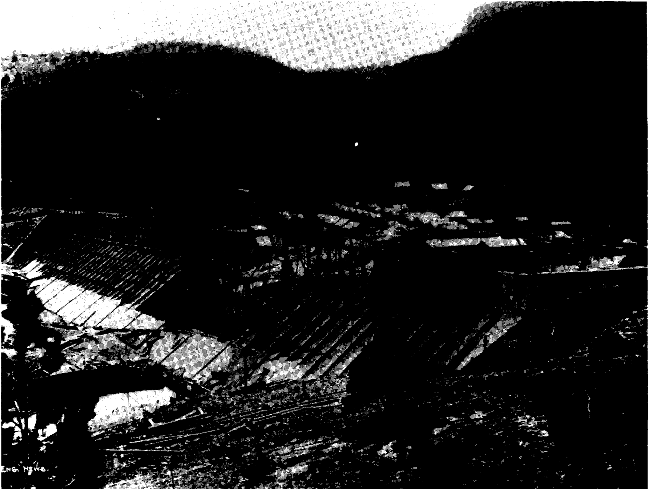
Figure 7. The Hauser Lake dam under construction, 1907. View from upstream, or water face. From Engineering News 58 (November 14, 1907): 507.
