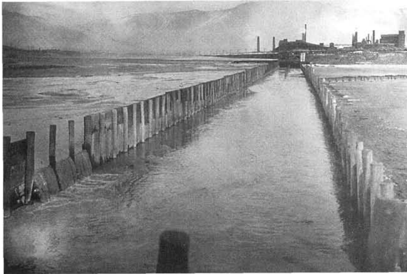
Figure 3. This photo, presented as evidence in 1905 in Magone v. Colorado Smelting and Mining Company, et al. , shows an open "culvert" carrying Silver Bow Creek through the tailings impoundments at the Butte Reduction Works at Butte, Montana. Water flowing into the culvert on the left is the overflow from an impoundment where solid tailings have settled after having been discharged from the concentrator at the smelter; visible in the background. Such a technology for managing industrial wastes would not normally have attracted the attention of a photographer; had it not been for the trial. Photo courtesy of the National Archives, Seattle Branch.
