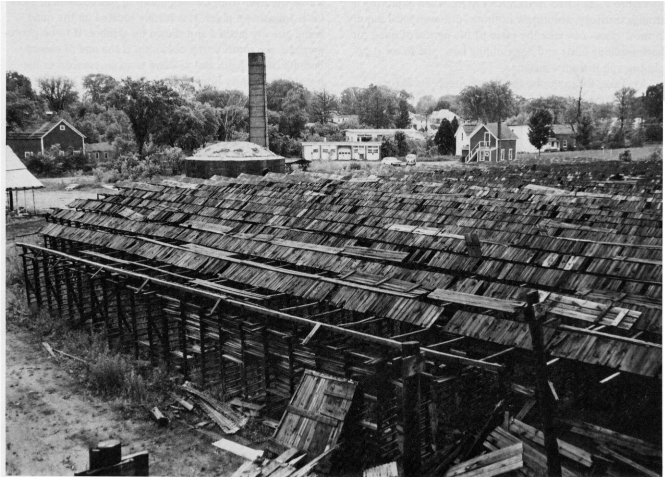
Racks for air-drying green brick, and coal-fired beehive kiln (1920s?), Drury brick works. 1972
